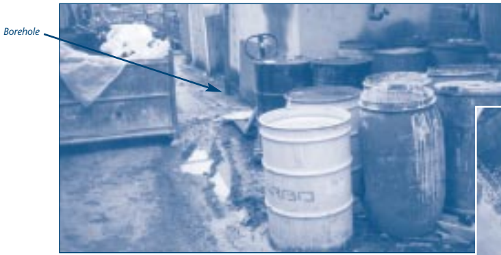
Storage of chemicals and fuels close to and up-slope of a borehole which is completed below ground, with no drain in manhole...
