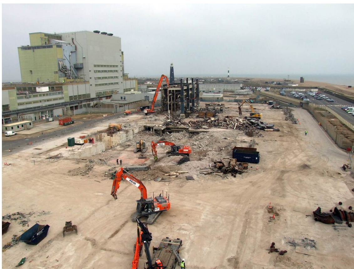
Dungeness A turbine hall demolition
