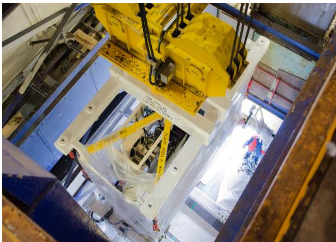
The arrival of a custom-built machine to scoop the radioactive contents from one of Sellafield's most hazardous buildings (Magnox Swarf Storage Silo).
