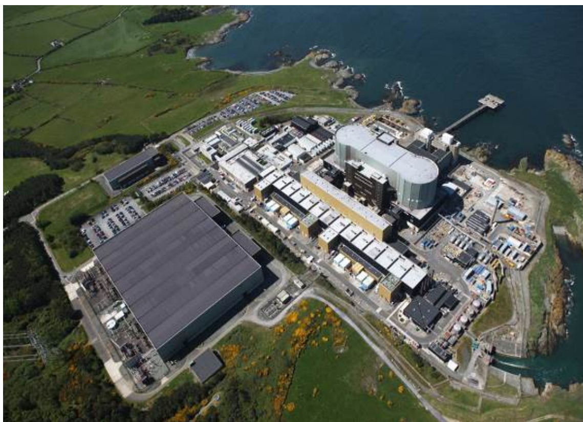
After a 5 year lifetime extension, Wylfa ceased generation in December 2015.
