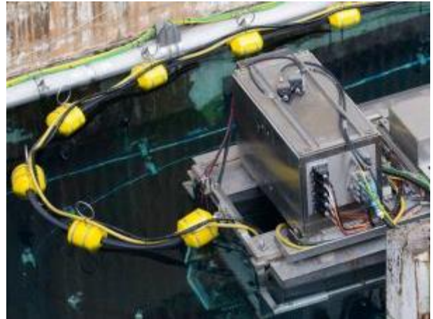
The first sludge retrievals from the pond
