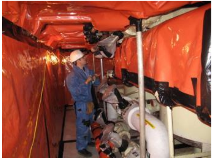
Asbestos removal at Chapelcross
