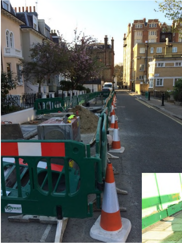
Single Lane working
