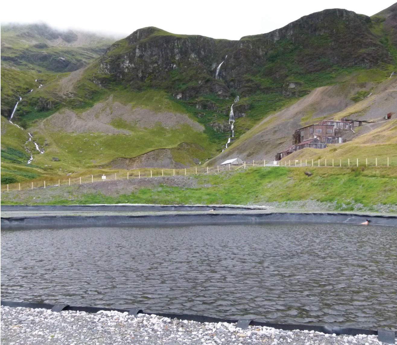
Mine water treatment lagoons at Force Crag.
