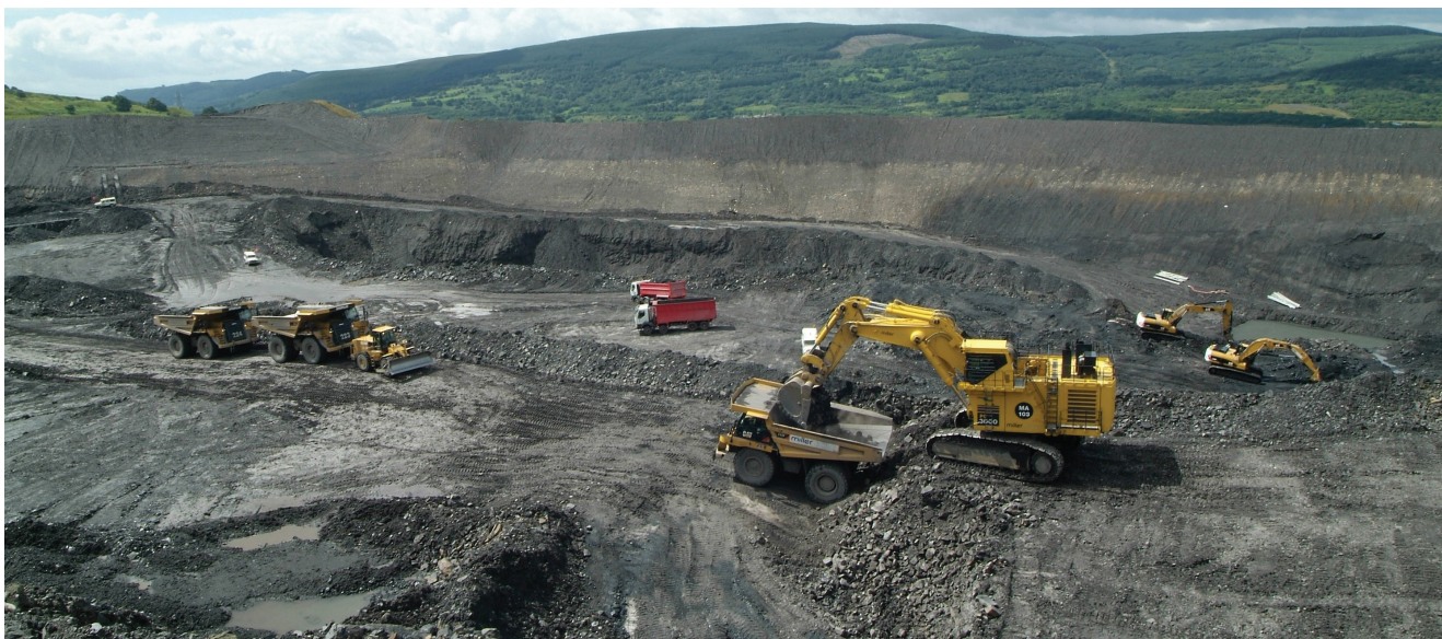
Ffos-y-Fran land reclamation scheme.
