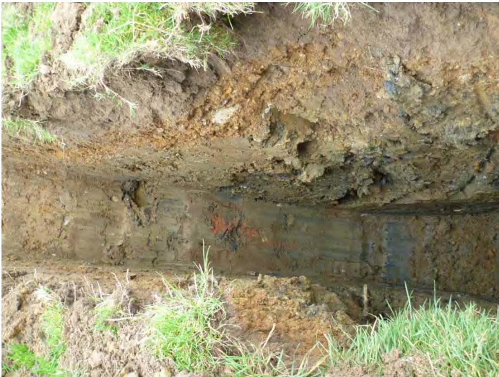
Plate 5 TP2 Topsoil overlying subsoil overlying Made Ground.
