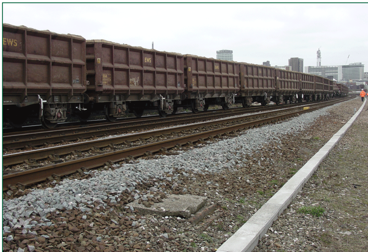
Figure 3: The incident site of the derailed wagons
