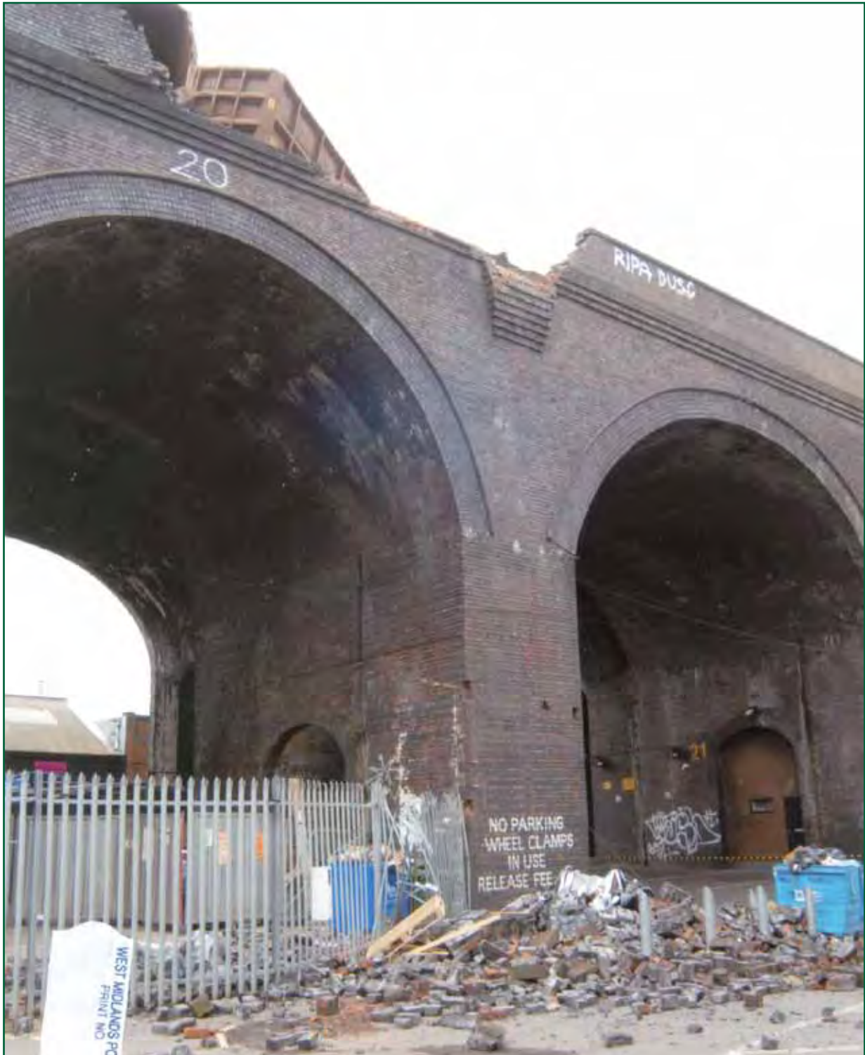
Figure 10: Fallen debris and damage to the parked car (image courtesy of West Midlands Police)
