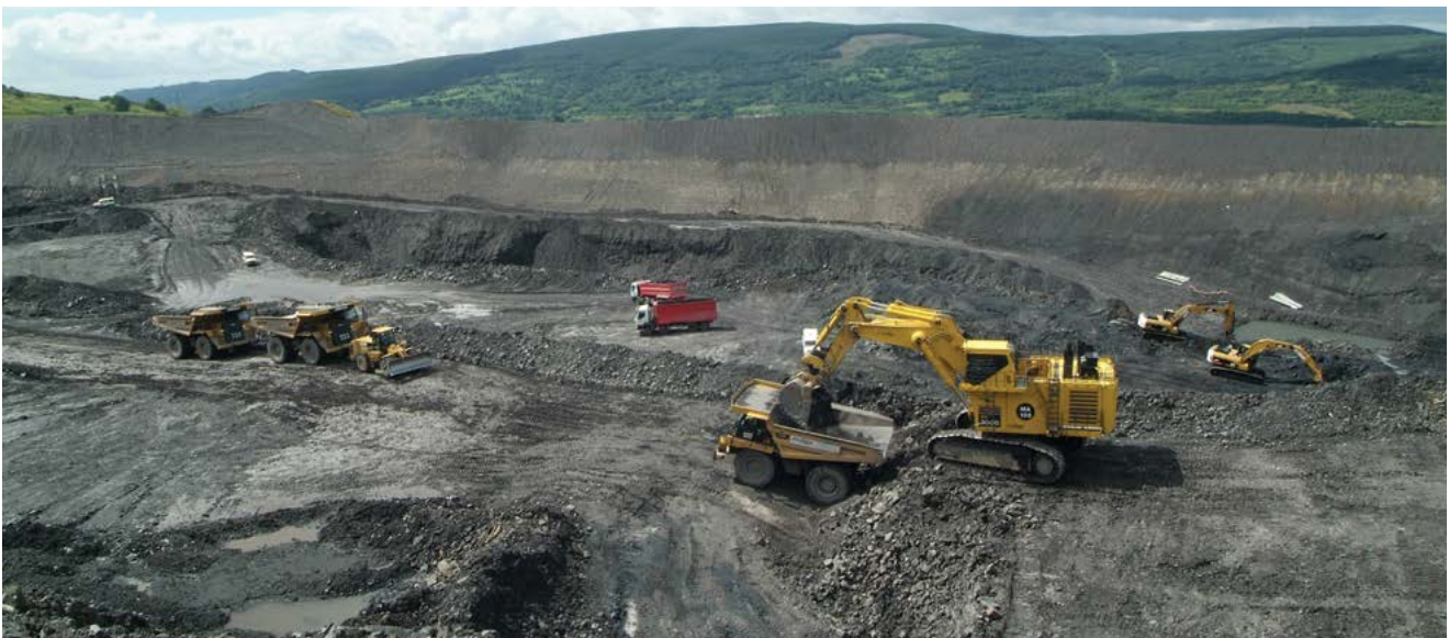
Ffos-y-Fran land reclamation scheme.
