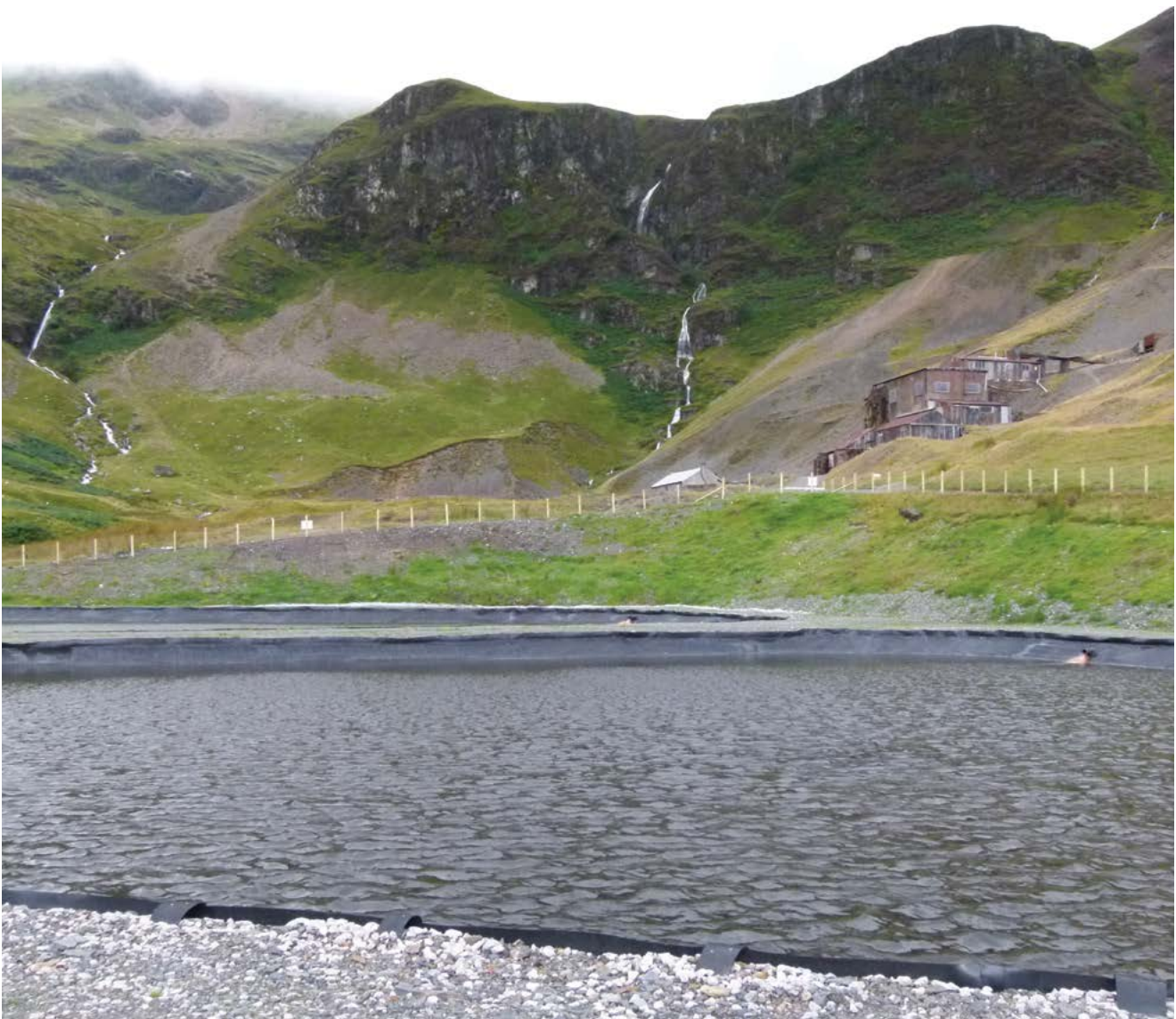
Mine water treatment lagoons at Force Crag.
