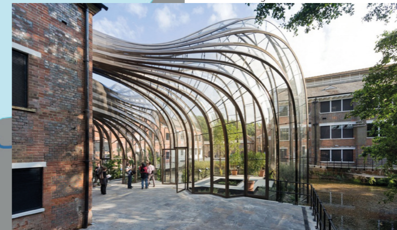
Old office buildings re-used as new work hubs
