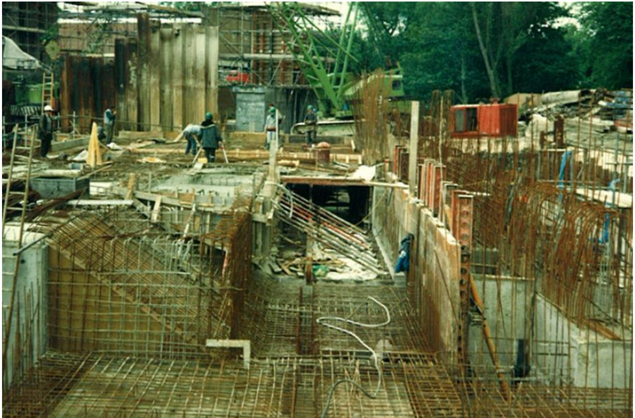
Construction Photograph 1. Downstream view, service tunnel within main building.
