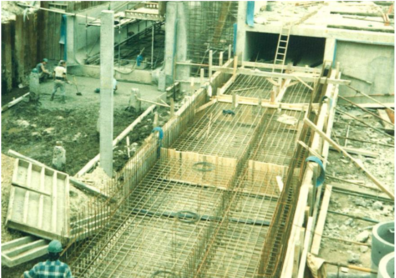
Construction Photograph 5. Upstream view, service tunnel within main building.
