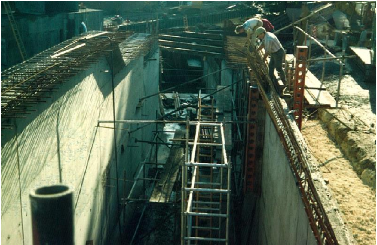
Construction Photograph 11. Downstream view, discharge culvert.
