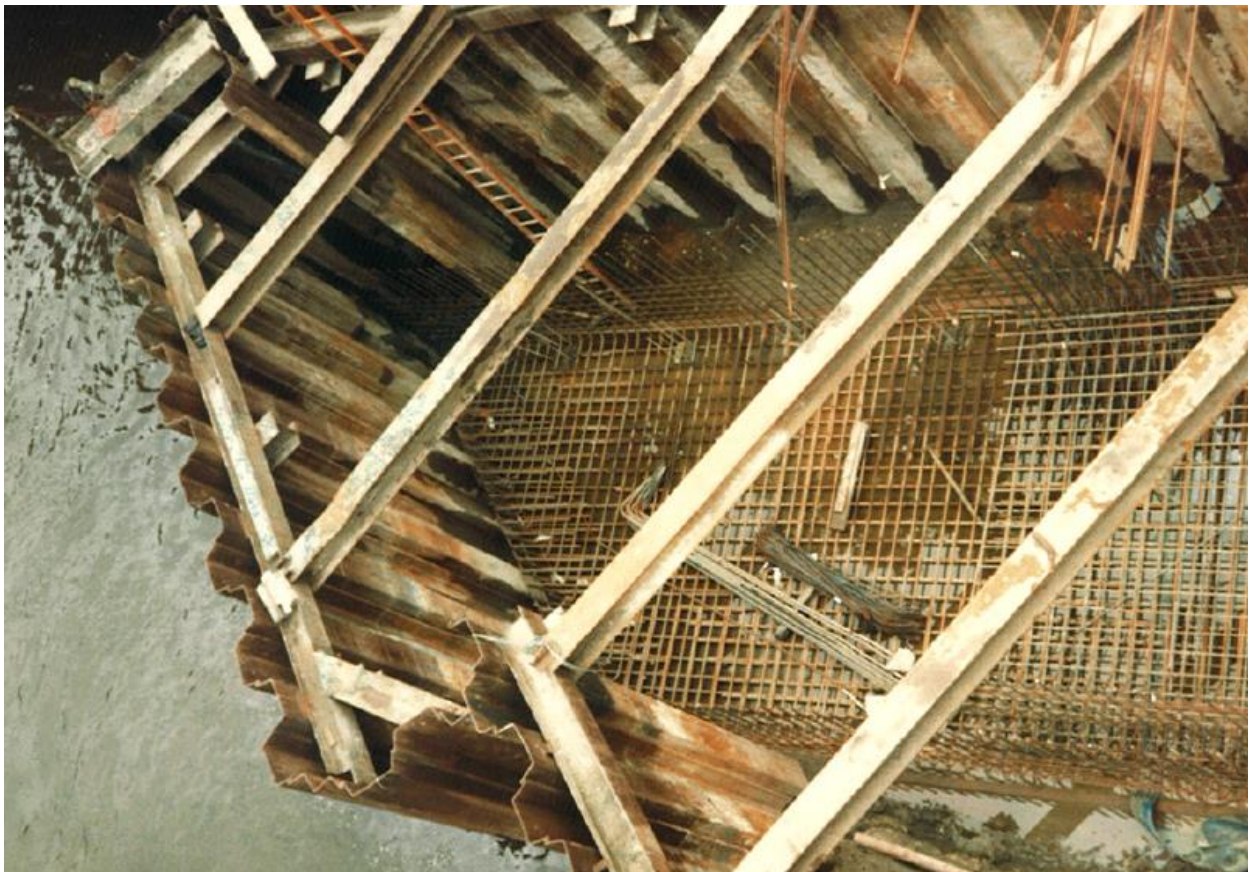
Construction Photograph 10. Discharge culvert.
