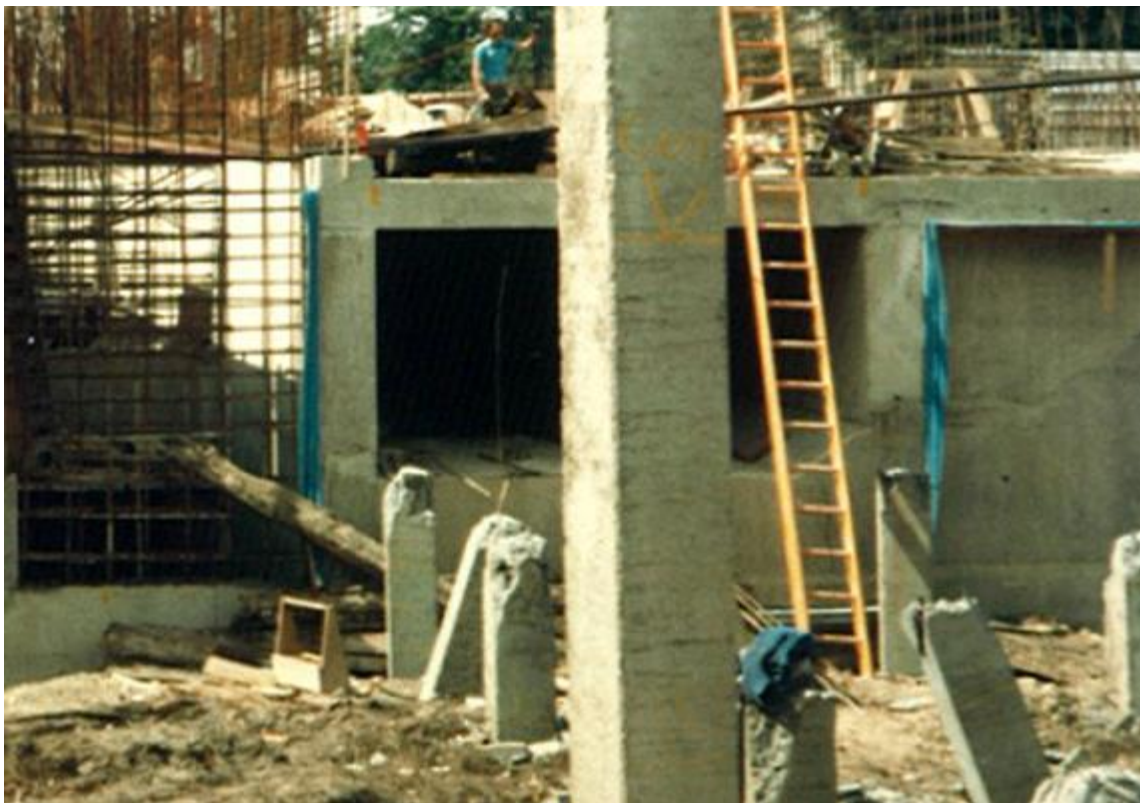
Construction Photograph 3. Upstream view, service tunnel within main building.
