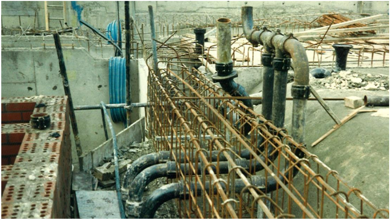
Construction Photograph 13. Interception chambers (left) and vents (x3) and building drainage.
