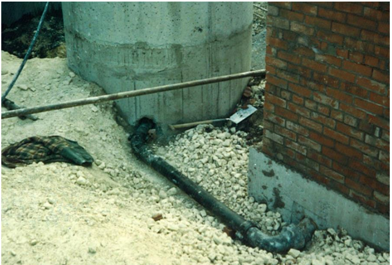
Construction Photograph 14. Interception chambers (right) and wet well.
