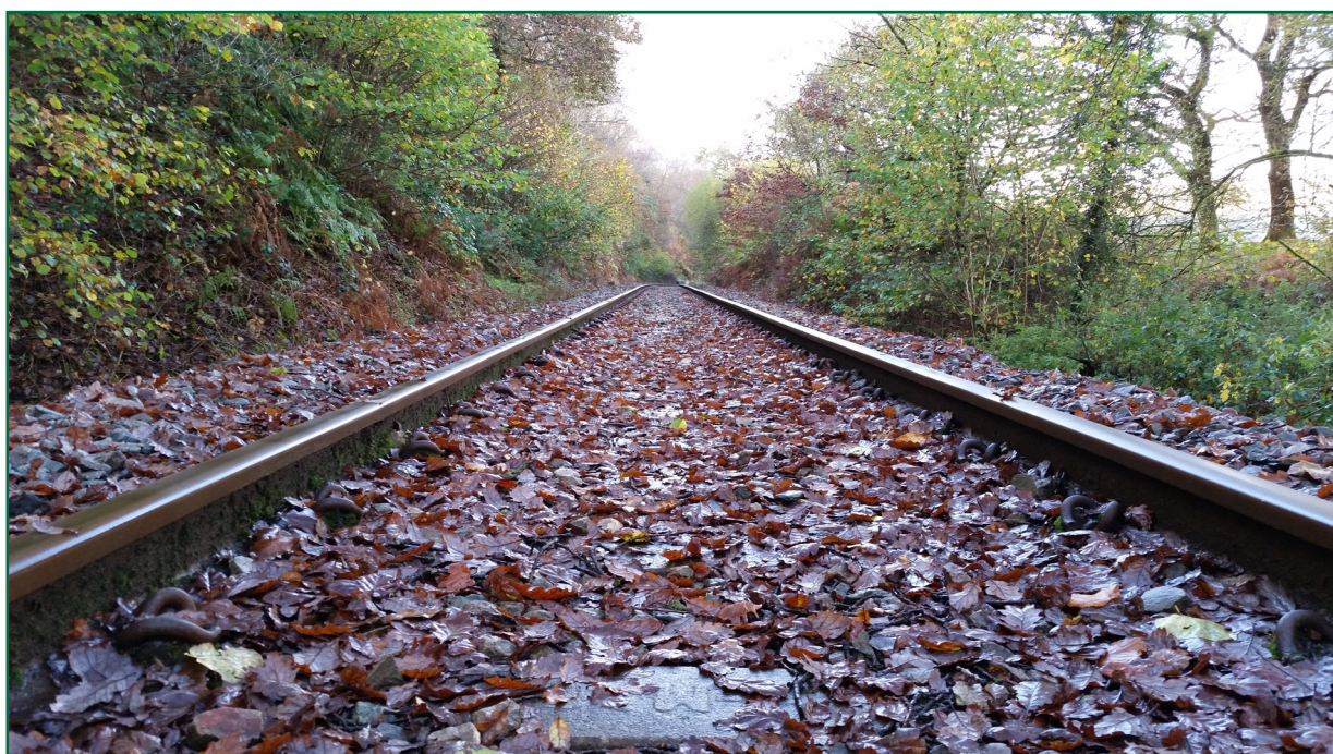
Figure 13: Garnant Branch line below GCG on 3 November 2014
