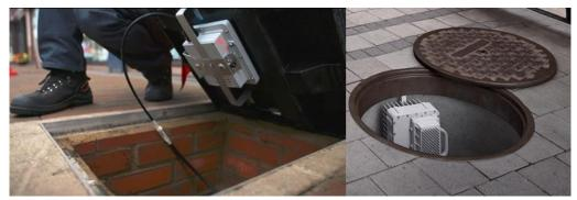
Figure 31: Pavement deployment of small cells. Source: 3G4G Small Cells Blog 68
