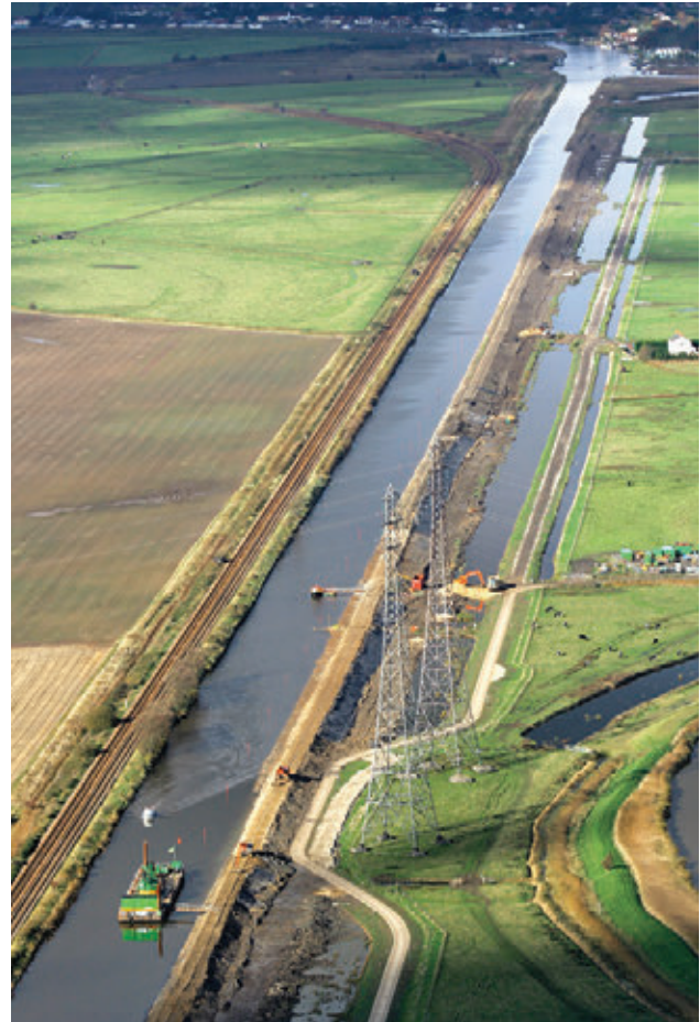
Flood bank construction, Haddiscoe Cut
