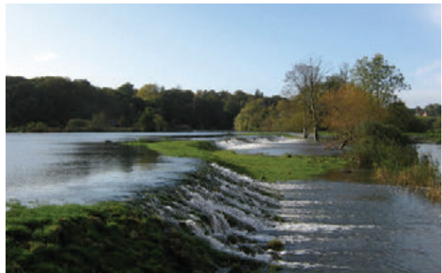
Overtopping at Postwick Marshes, River Yare
