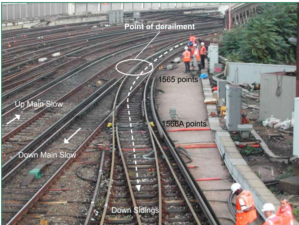
Figure 8: View of 1565 points looking towards London Waterloo, showing route of train 5G05
