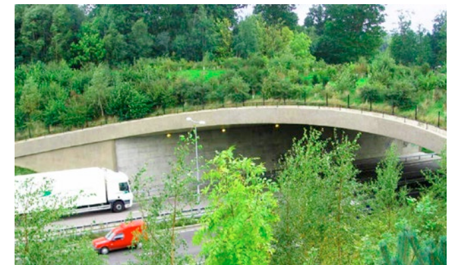
Illustration from the HS2 Landscape Design Approach document - A21 Lamberhurst Bypass land bridge.
