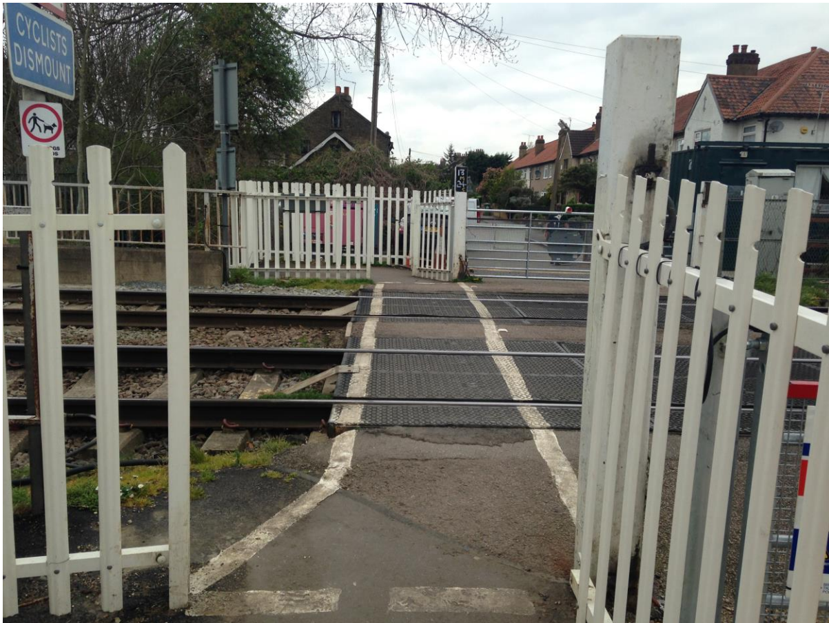
Trinity Lane footpath crossing (image courtesy of Network Rail)
