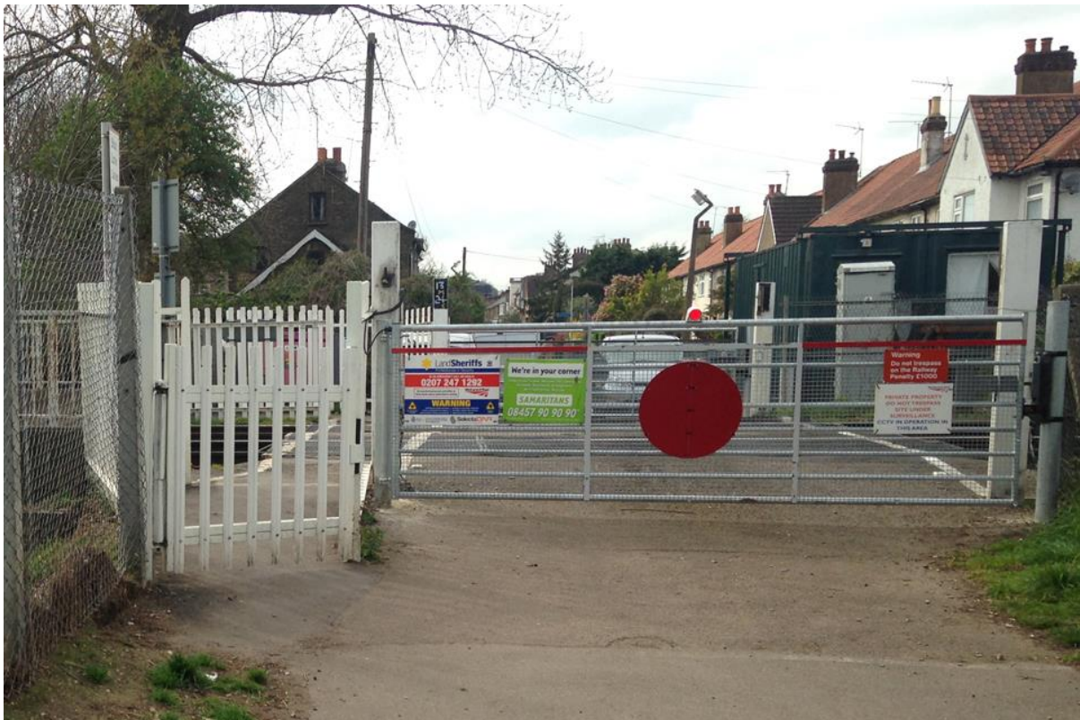
Trinity Lane footpath and vehicle level crossings, from the east (image courtesy of Network Rail)
