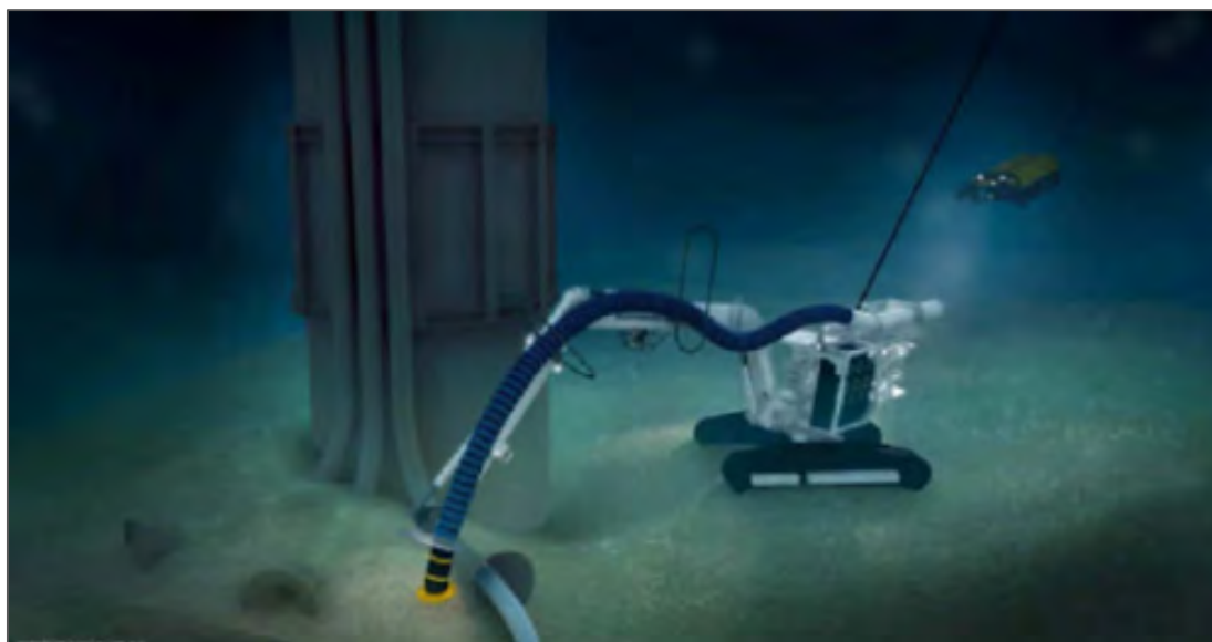
Figure 9-8: Using a Subsea Dredger to Excavate a Pit
