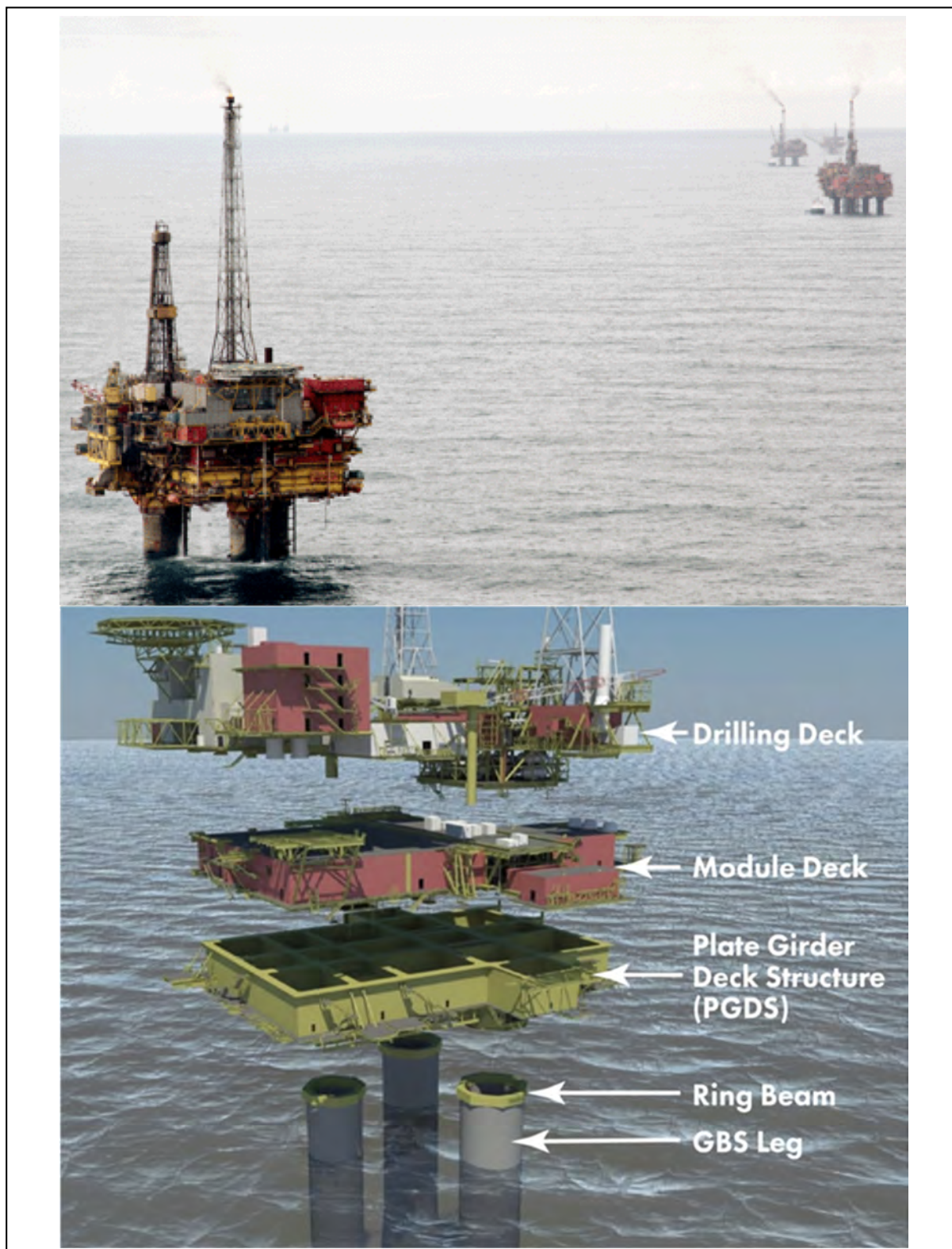
Figure 8-4: Brent D Topsides General Configuration
