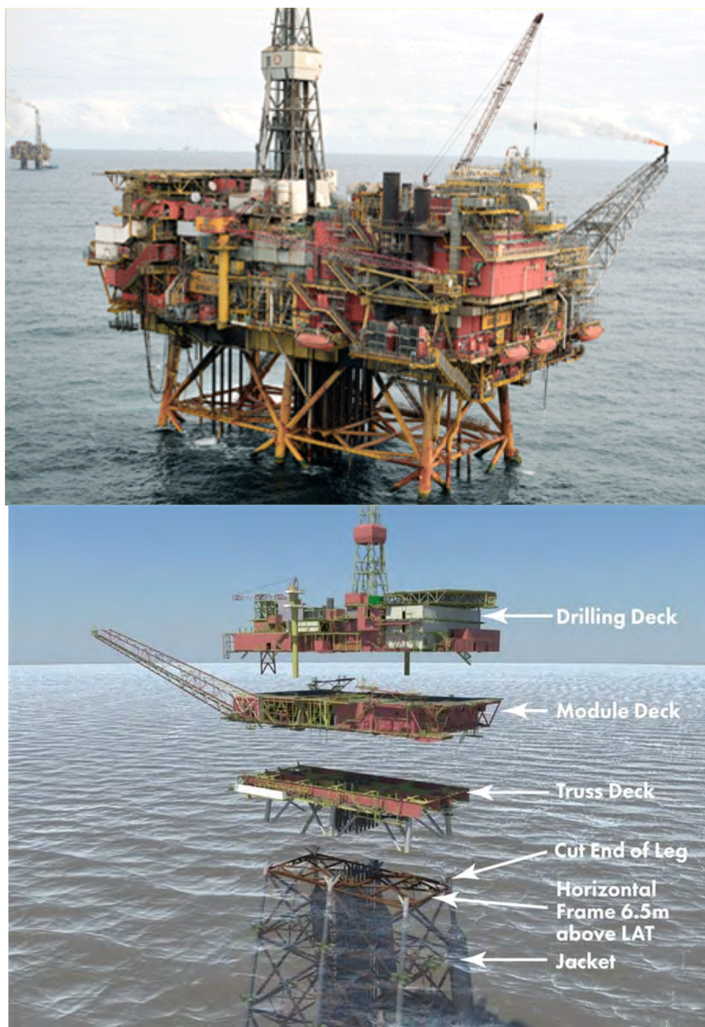
Figure 8-1: Brent A Topsides General Configuration
