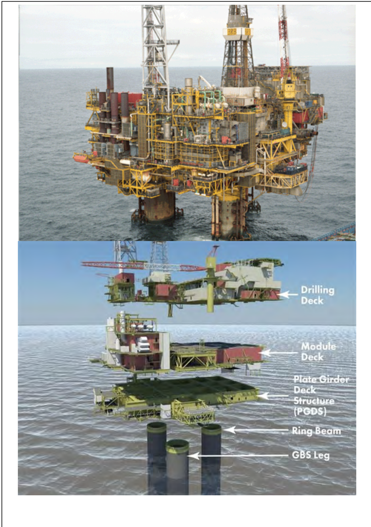
Figure 8-2: Brent B Topsides General Configuration
