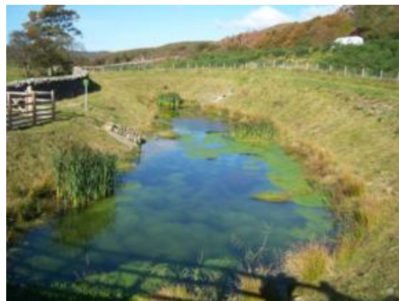
Figure 9.26 – OYA - Barrows Green balancing pond with marginal planting beginning to establish. Algae noticeable within the water body
