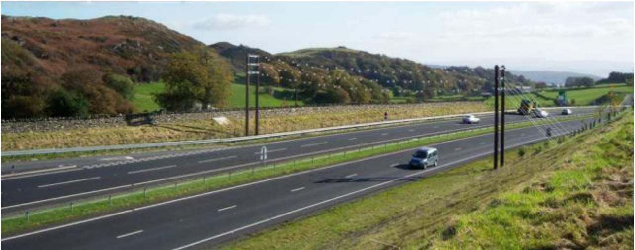
Figure 9.14 – OYA - View to bat guidance structure provided across the bypass near Low Newton
