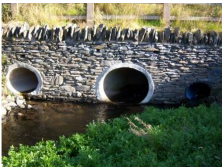
Figure 9.20 – OYA - Culvert and mammal tunnel below bypass at Belman Beck
