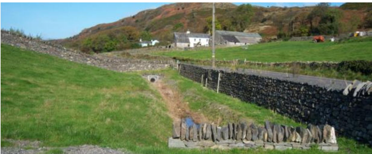
Figure 9.24 - Example of toe of embankment drainage ditch with local stone clad headwall
