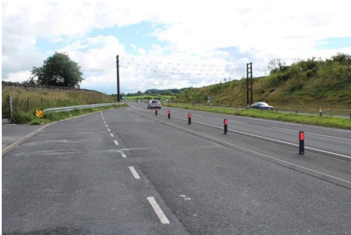
Figure 9.15 - FYA – Adjacent planting is beginning to establish although not yet mature enough to guide bats to closely link to the guidance structure
