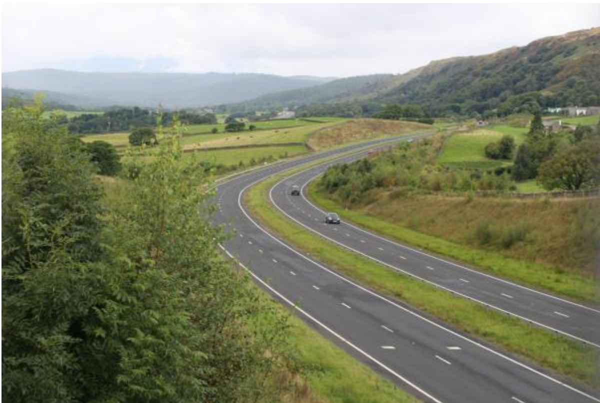
Figure 9.8 - FYA September 2013 - illustrating typical good growth within planting plots. Oak Head cutting slopes visible to right with Meadow Croft cutting in middle distance.
