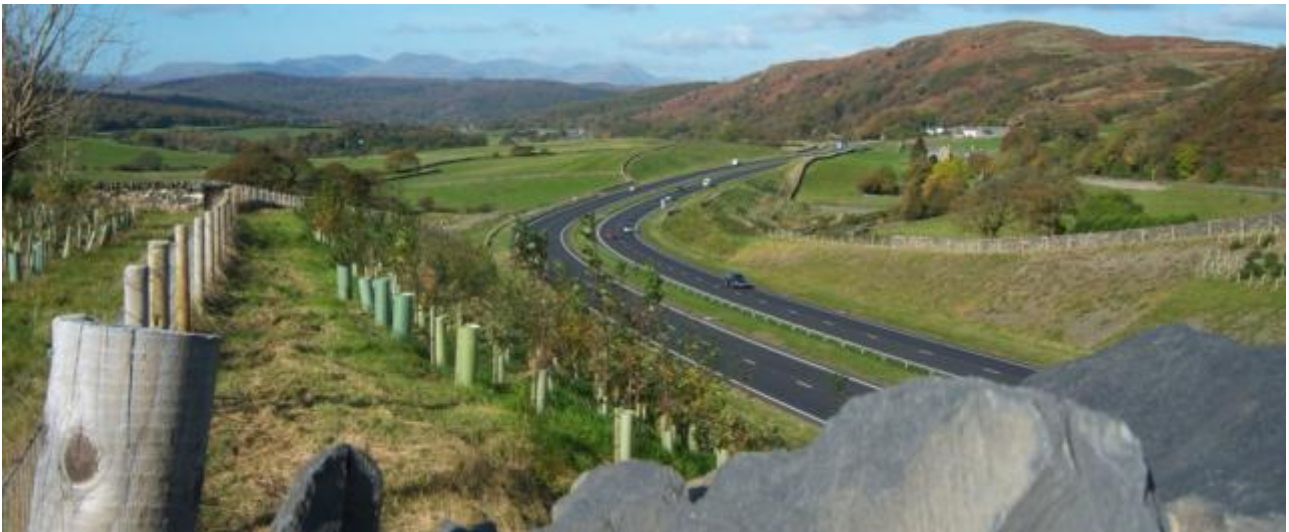
Figure 9.7 – OYA - View west from Head House Road over-bridge
