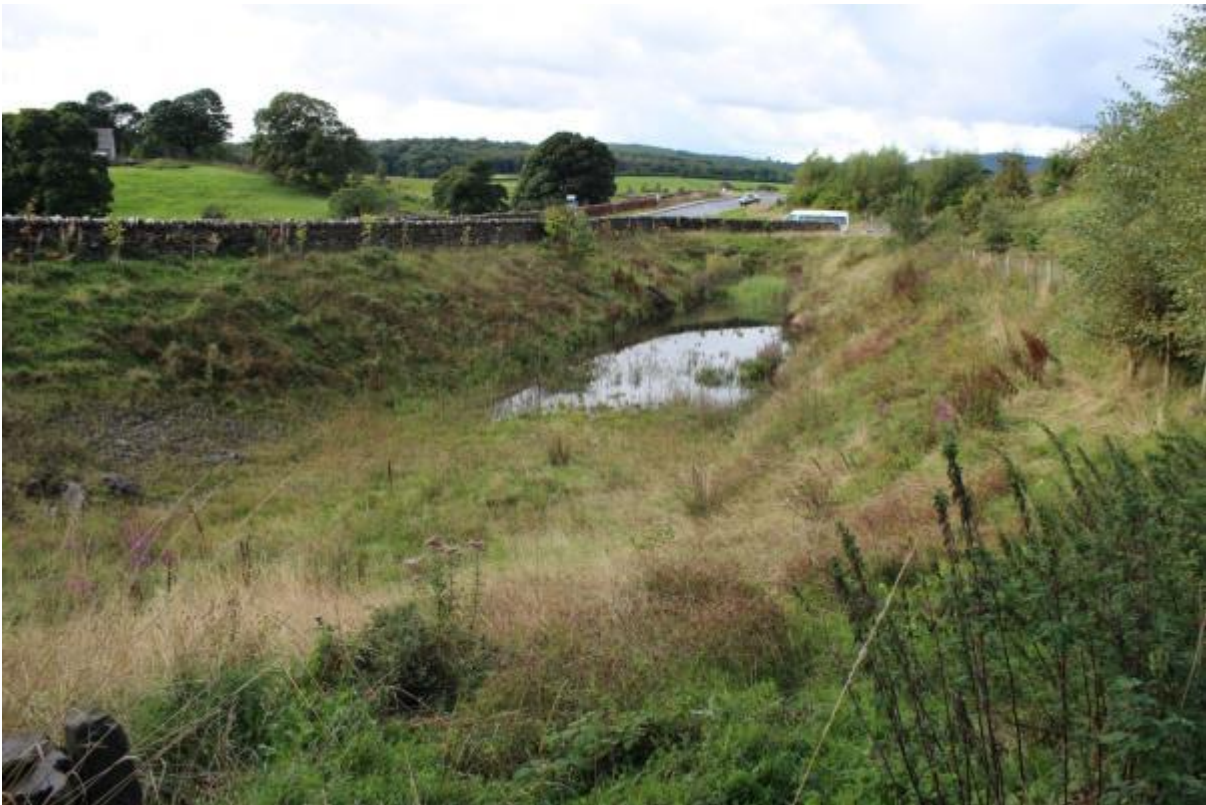
Figure 9.24 - Example of toe of embankment drainage ditch with local stone clad headwall
