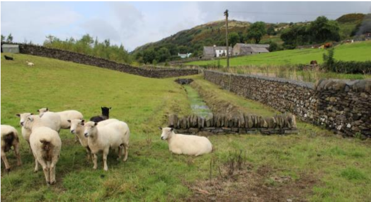
Figure 9.26 – OYA - Barrows Green balancing pond with marginal planting beginning to establish. Algae noticeable within the water body
