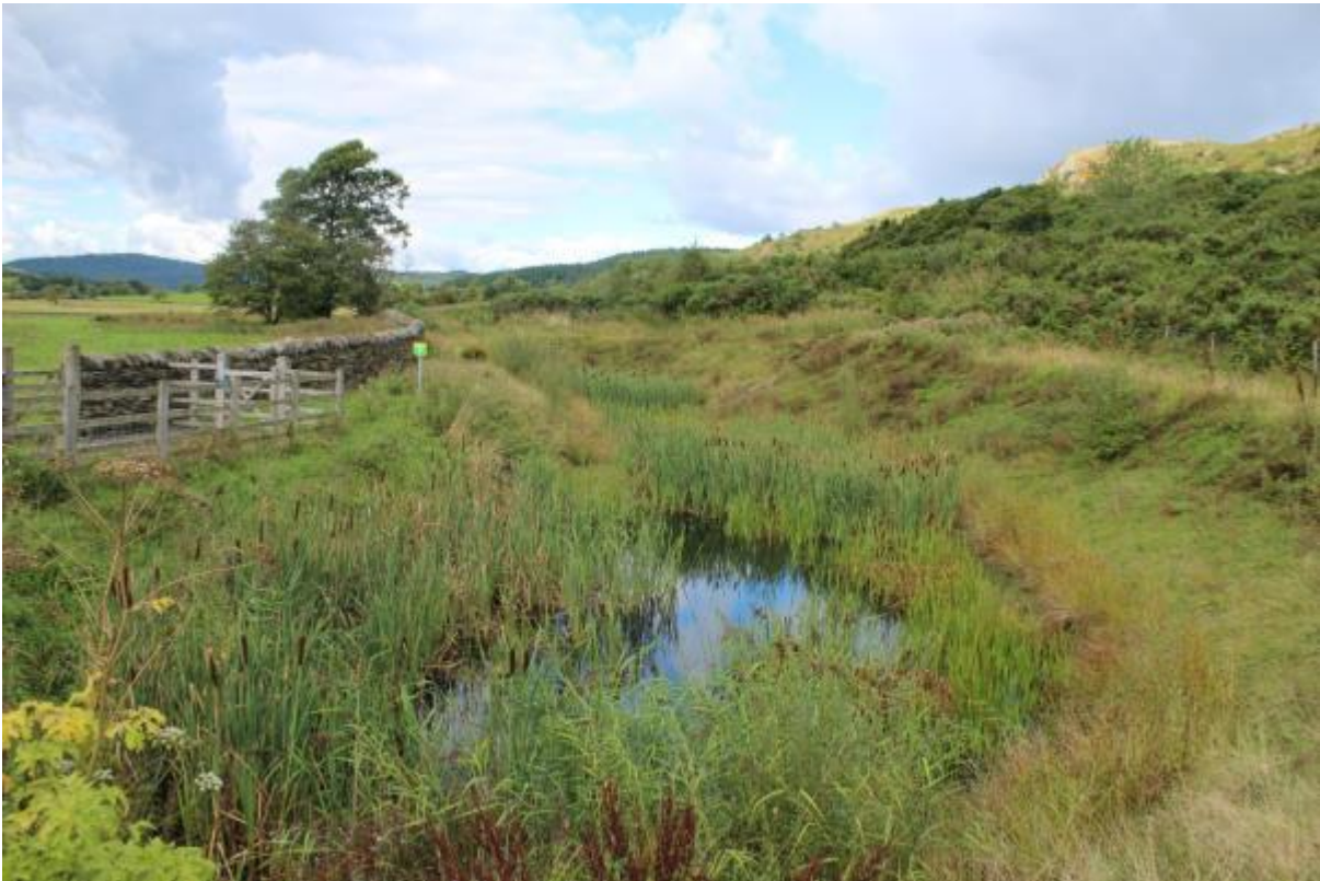
Figure 9.27 - FYA September 2013 – the balancing pond has a balance of open water and marginal vegetation. No algae was present
