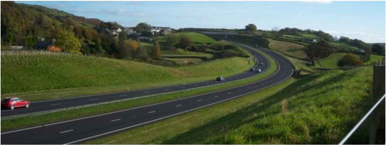
Figure 9.9 – OYA – View east towards Head House over-bridge and High Newton to left. Curved alignment avoids ‘notch’ effect of road cutting through hillside
