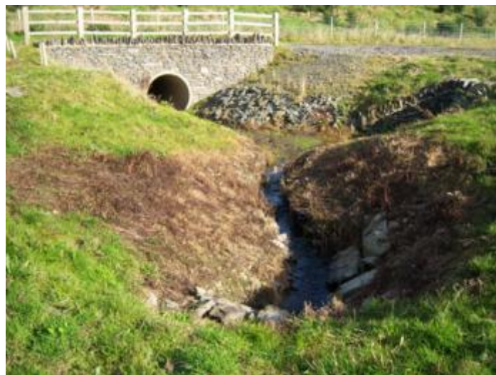
Figure 9.28 – OYA - Naturalistic realignment of Newton Beck which has been culverted under the bypass
