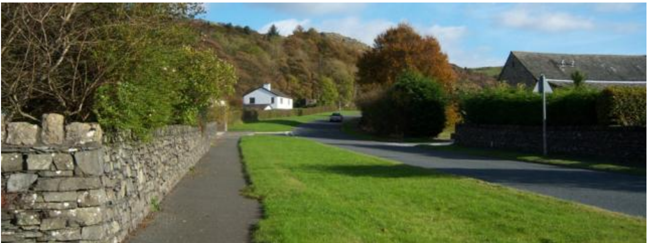
Figure 5.8 – Old A590 in High Newton with reduced carriageway and widened verge
