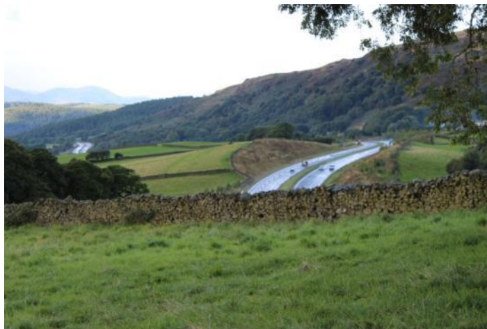
Figure 5.5 - View from lane near Head House over-bridge looking west illustrating bypass alignment curving within the local landscape to minimise impact on the high quality National Park landscape
