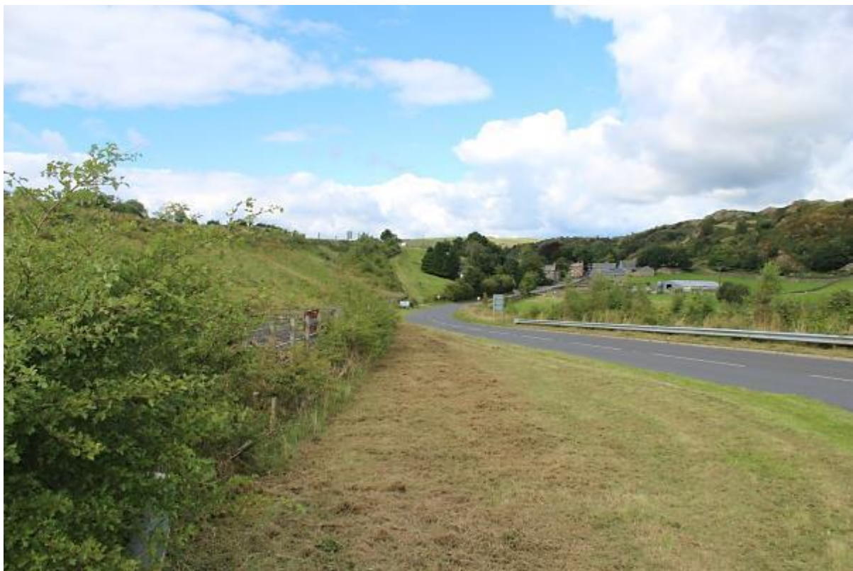
Figure 9.6 - FYA September 2013 – hedge generally establishing well although some areas exhibit slower growth. Triangular fenced plot in centre view is establishing as expected for FYA planting. Planting on the main embankment slope is slow to establish and has yet to provide any screening or integration of the Cartmel junction.
