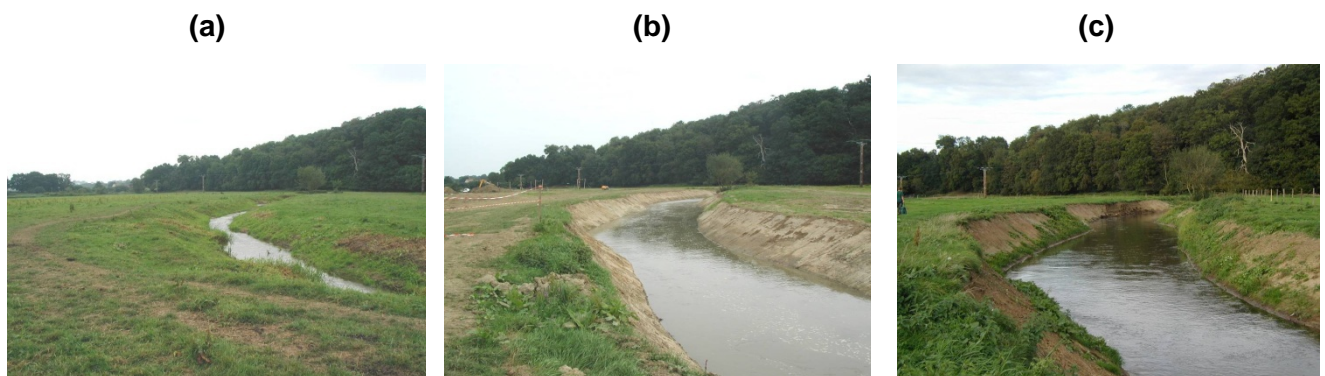
Figure 3.3 Meander loop (a) pre-restoration, (b) immediately post-restoration and (c) in 2007 three years post-restoration
