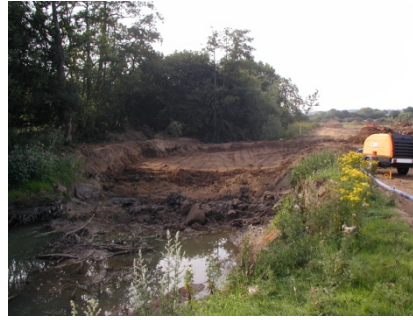
Figure 3.7 Construction of bund in canal cut
