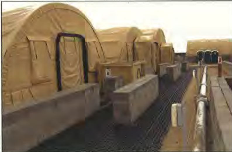
Fig 30. Tented accommodation in the COB. The exterior breezeblock blast protection was repeated inside the tents (Op Stonehenge).
