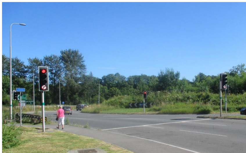
Figure 7-1 New Signals on the A345 North (Adjacent to the Subway)
