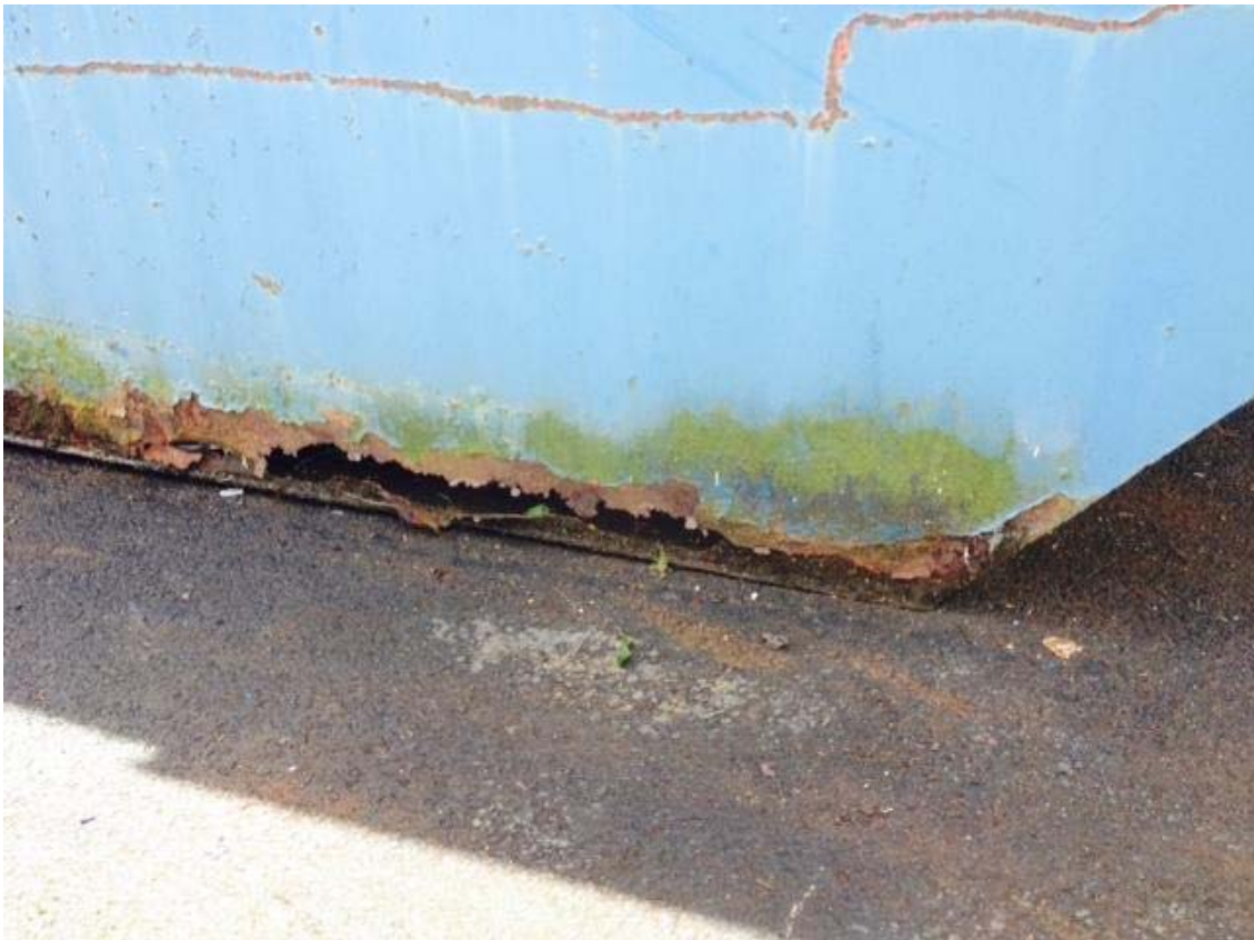
Figure 1 showing extensive corrosion
