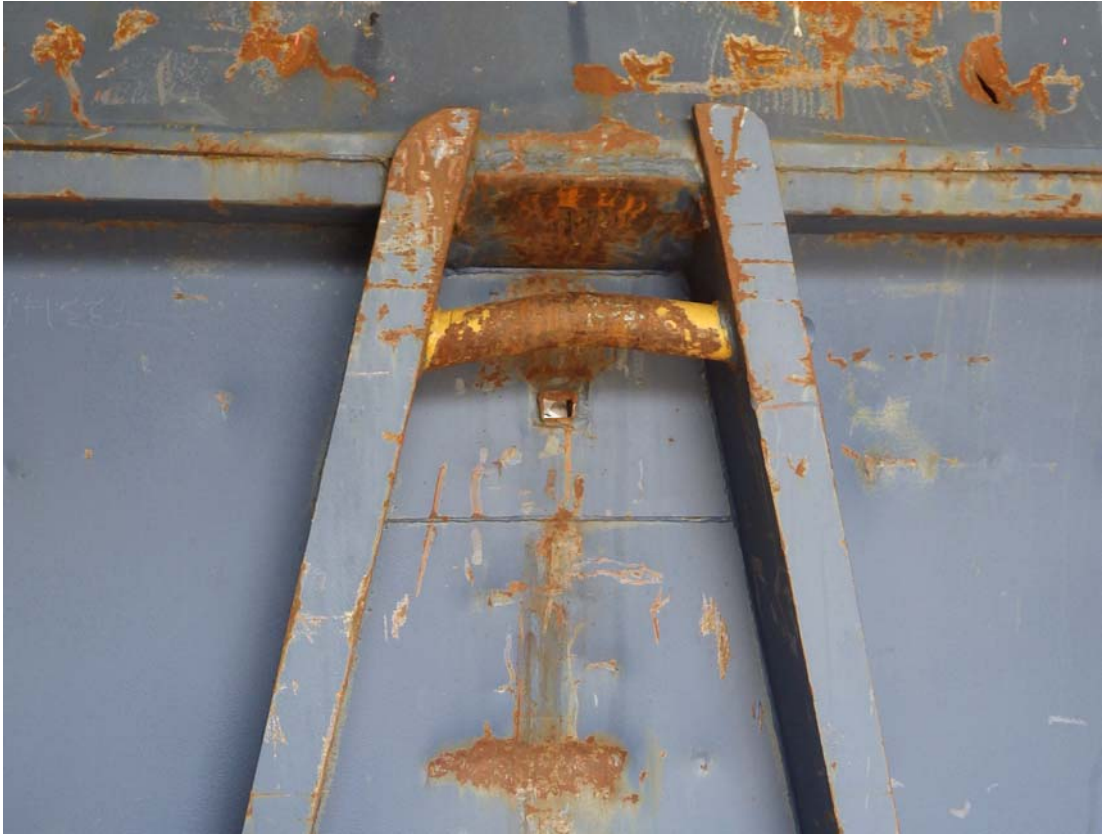
Figure 5 showing deflector plate positioned above bale bar preventing incorrect engagement
