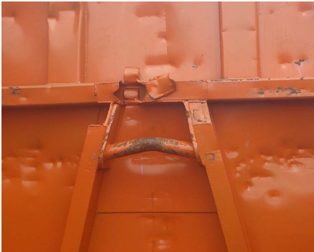
Figure 6 showing missing deflector plate and damage due to incorrect engagement
