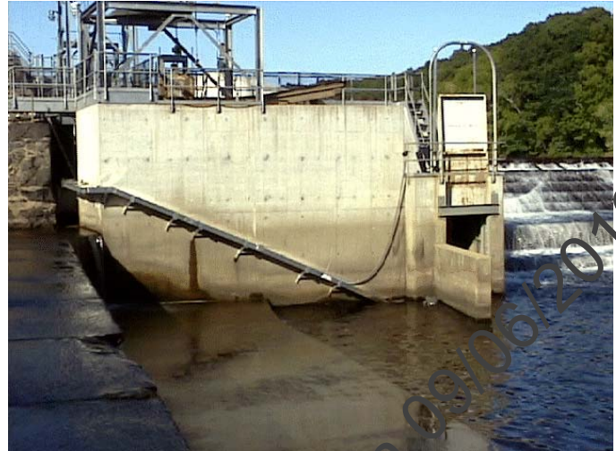
Figure 6.10. Eel pass-trap at Greenville Dam. Photograph Alex Haro
