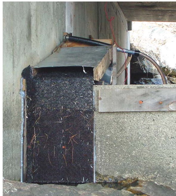
Figure 6.19. Vertical substrate board on the west ramp at West Harbor Pond. Photograph G. Wippelhauser.
