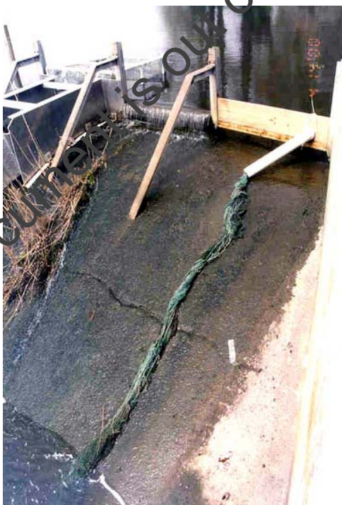
Left: Figure 6.17. Elver pipe-pass at Garrison Lake, Delaware, soon after installation. Photograph S Shotzberger.
