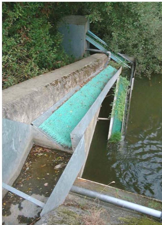
Figure 6.3. Upstream pass and pass-trap at Pont-es-Omnès
