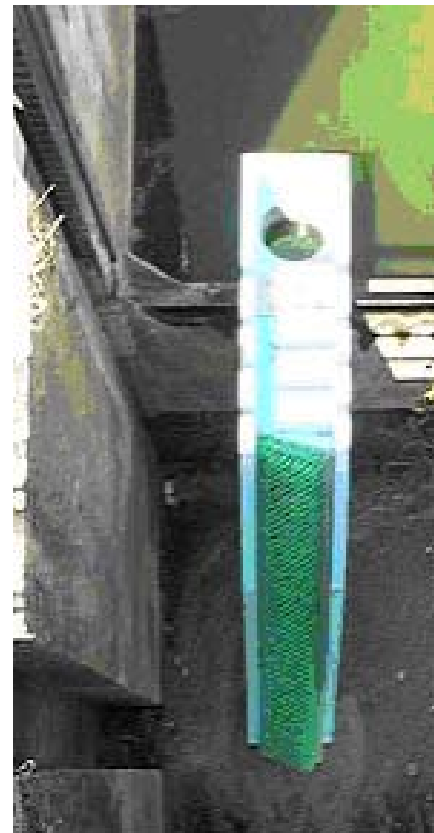
Figure 6.15. “Fish-Pass” prefabricated sluice-gate pass.
