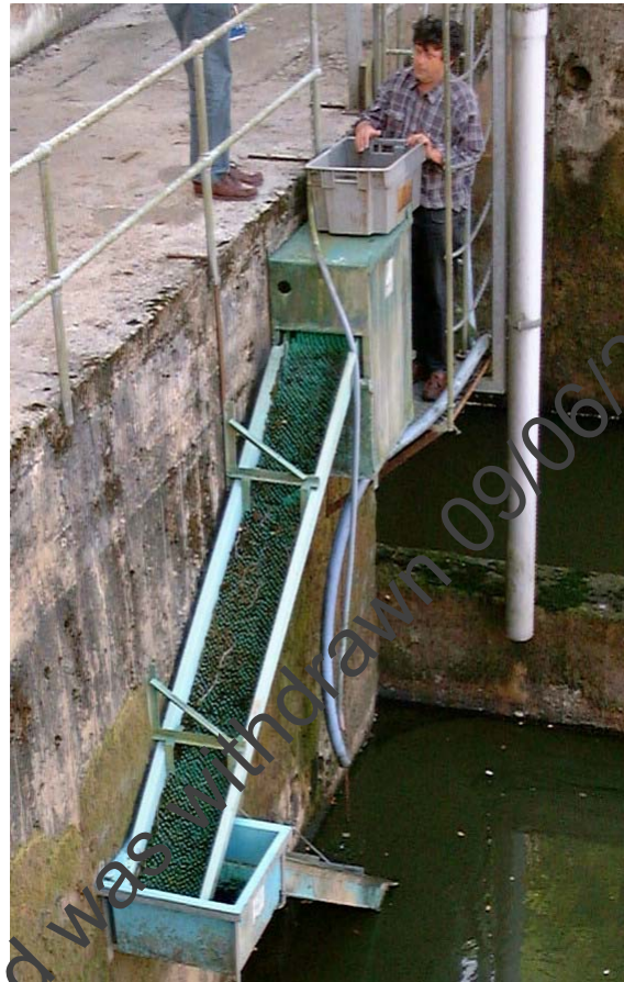
Figure 6.9. Rophemel Dam eel pass-trap.
