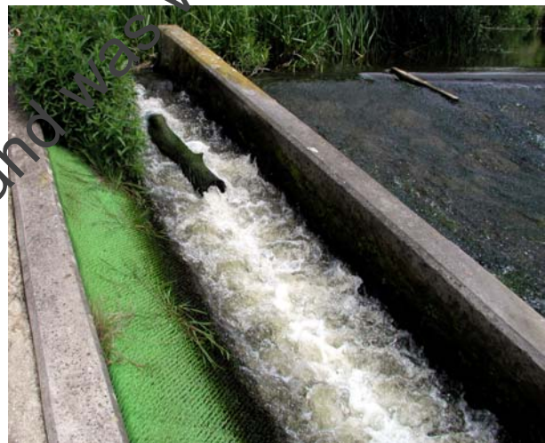
Figure 6.4. Eel pass at Chadbury
