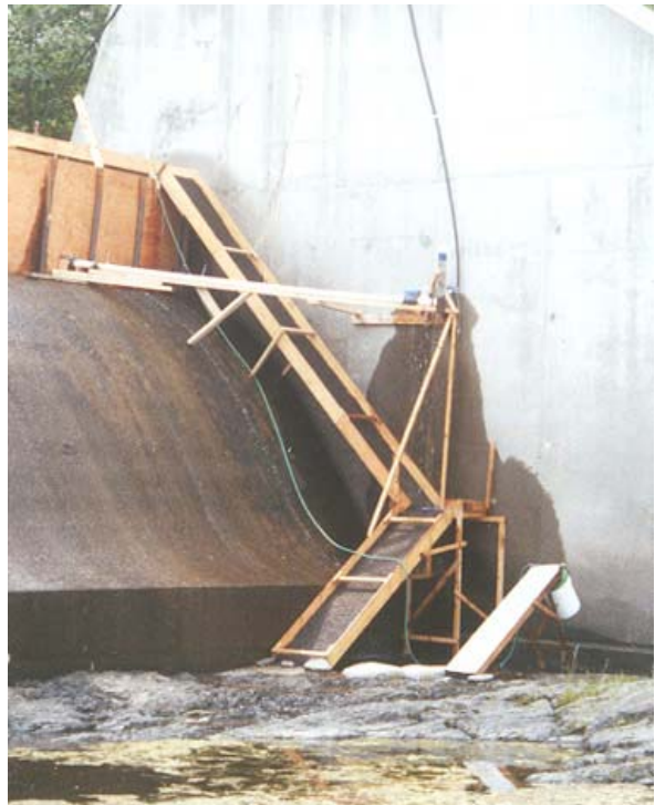
Figure 6.6. Pumped-supply pass at Fort Halifax Dam. A “portable passage” ramp (see Section 6.6.4) is being deployed alongside. Photograph G Wippelhauser.
