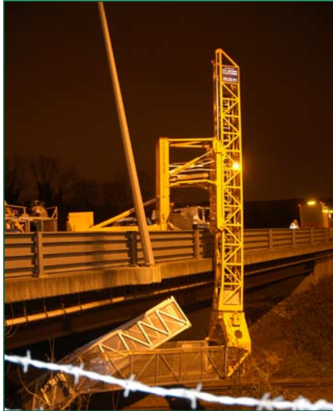
Figure 3: 'Moog' bridge inspection gantry viewed from motorway level after the collision (Photograph courtesy of the British Transport Police)
