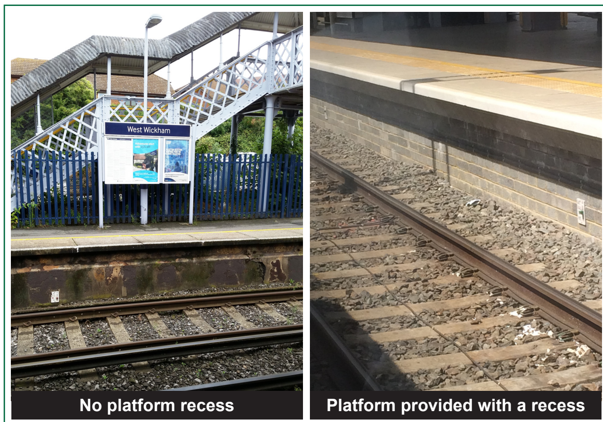
Figure 15: Recess providing survival space beneath platform
