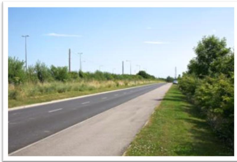
Figure 5.17 – Extensive hedgerow planting along the Elton link road (left) linked to the existing mature hedgerow (centre right), screening A66 traffic from the wider landscape and integrating the link road into the existing landscape framework
