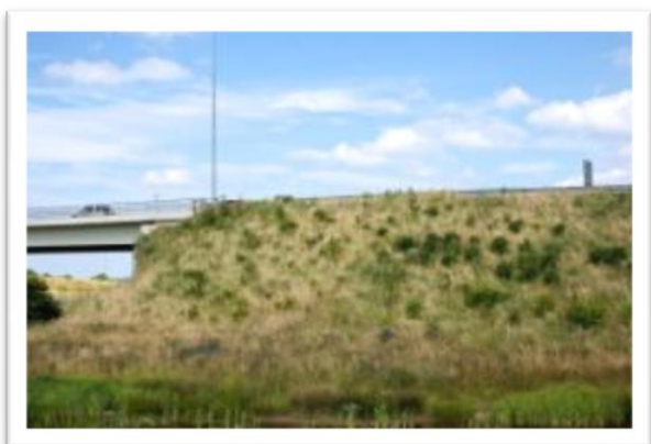
Figure 5.13 – Sparse/ stunted woodland planting on the west embankment of the GSJ
