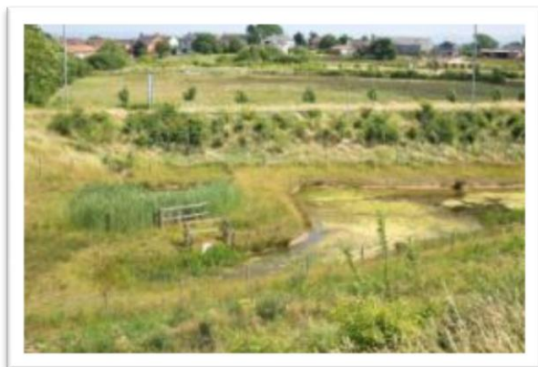
Figure 5.28 – Balancing Pond adjacent to the westbound carriageway
