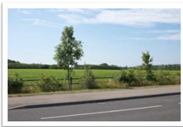
Figure 5.10 – Gaps in the hedgerows along the Elton link road at the eastern extents of the scheme
