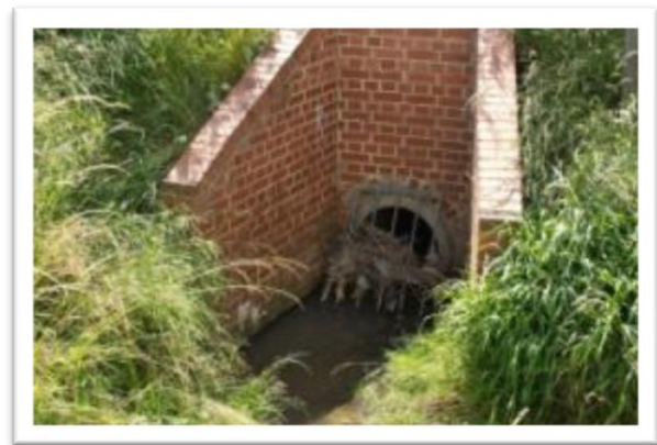
Figure 5.25 – Vegetation encroachment and the beginnings of grille blockages at Balancing Pond Inlets/ Outlets
