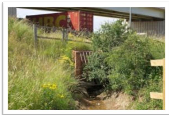
Figure 5.25 – Vegetation encroachment and the beginnings of grille blockages at Balancing Pond Inlets/ Outlets
