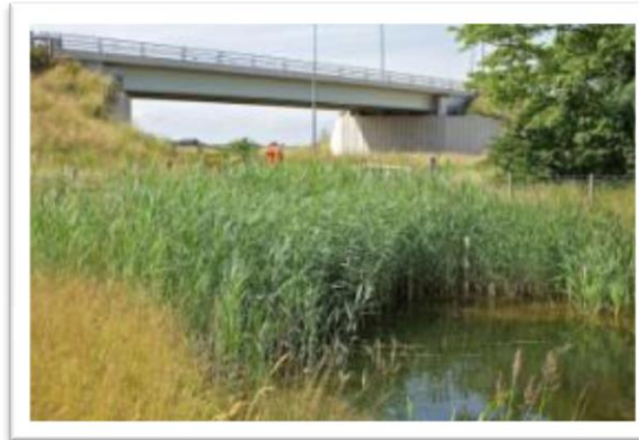
Figure 5.20 – Balancing pond with well established marginal planting
