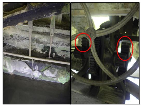
View (L) of the twin controls to the turbine inlet sluices. The inlet sluices are raised and lowered by turning the wheel at the top of the mechanism (R). The position of both sluices can be seen to be almost closed (red circles).
