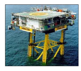
These platforms are two-level, normally unmanned structures with an underdeck. Produced gas, together
