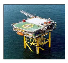
Lennox produces both gas and condensate, together with formation water. These reservoir fluids are routed to the Douglas Complex for separation. Lennox lies approximately 8 km off the Sefton coast. The Lennox Platform is a two level, 12 well slot structure with an underdeck. Water depth at the location is 7m.
