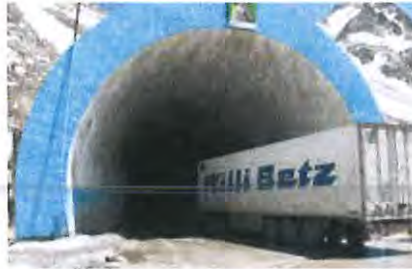
The entrance to the Salang Pass Tunnel
