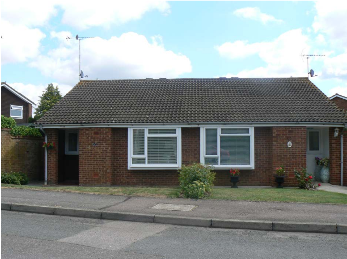
Source: BRE photo library
