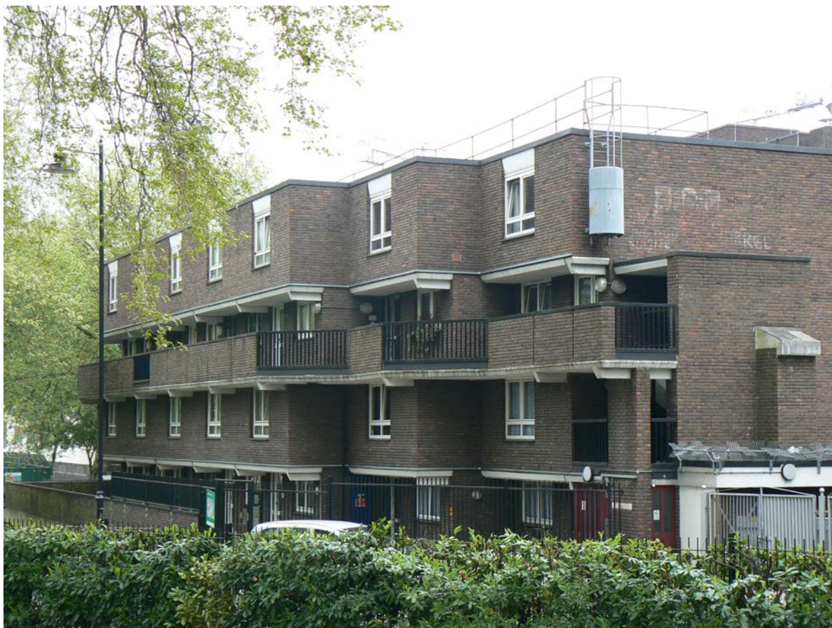
Source: BRE photo library
