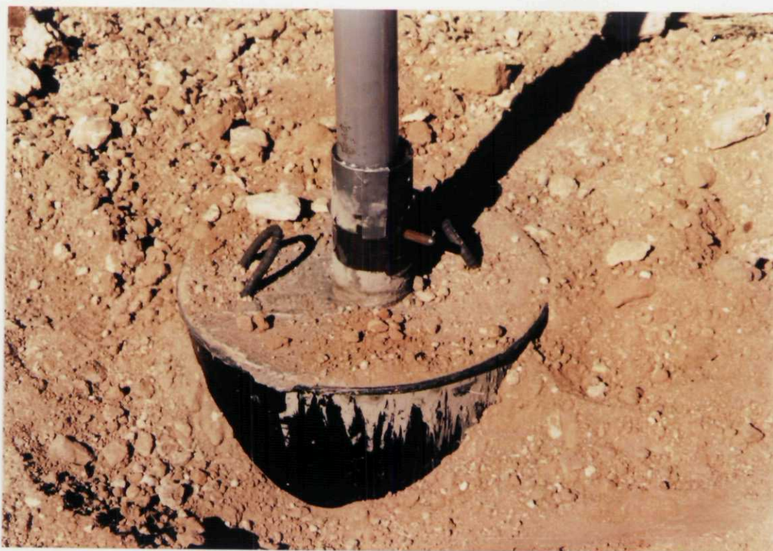
Figure 19. Buried concrete drums provide support for sign posts
