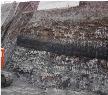
Excavated Cutting Slope
