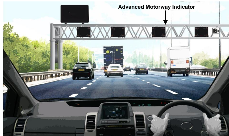
Figure 4A: Illustrative M6 Junction 16 to 19 Smart Motorway All Lane Running scheme section operating in normal motorway conditions with blank advanced motorway indicators and blank gantry mounted variable message sign
