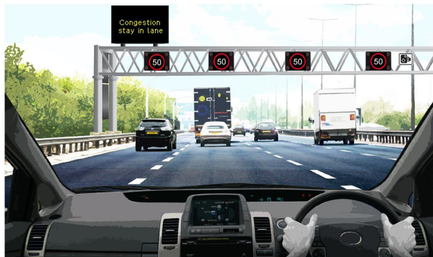
Figure 4C: Illustrative M6 Junction 16 to 19 Smart Motorway All Lane Running scheme section operating with variable mandatory speed limits
