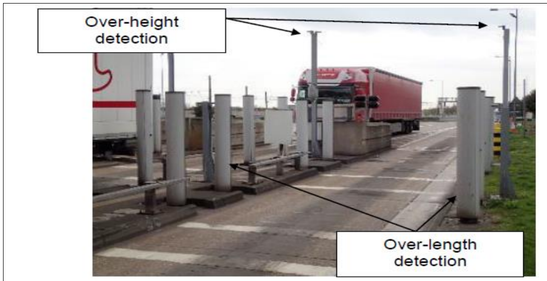
Figure 21: Over-length and over-height detection
