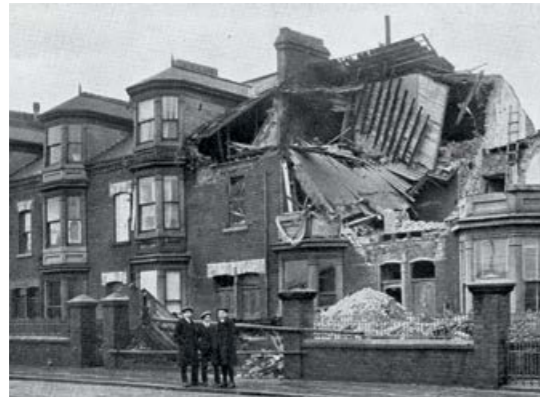
Damaged housing in Hartlepool following the German naval bombardment, December 1914 © IWM HU 12823
