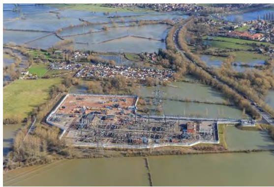
Walham with permanent protection 2013
