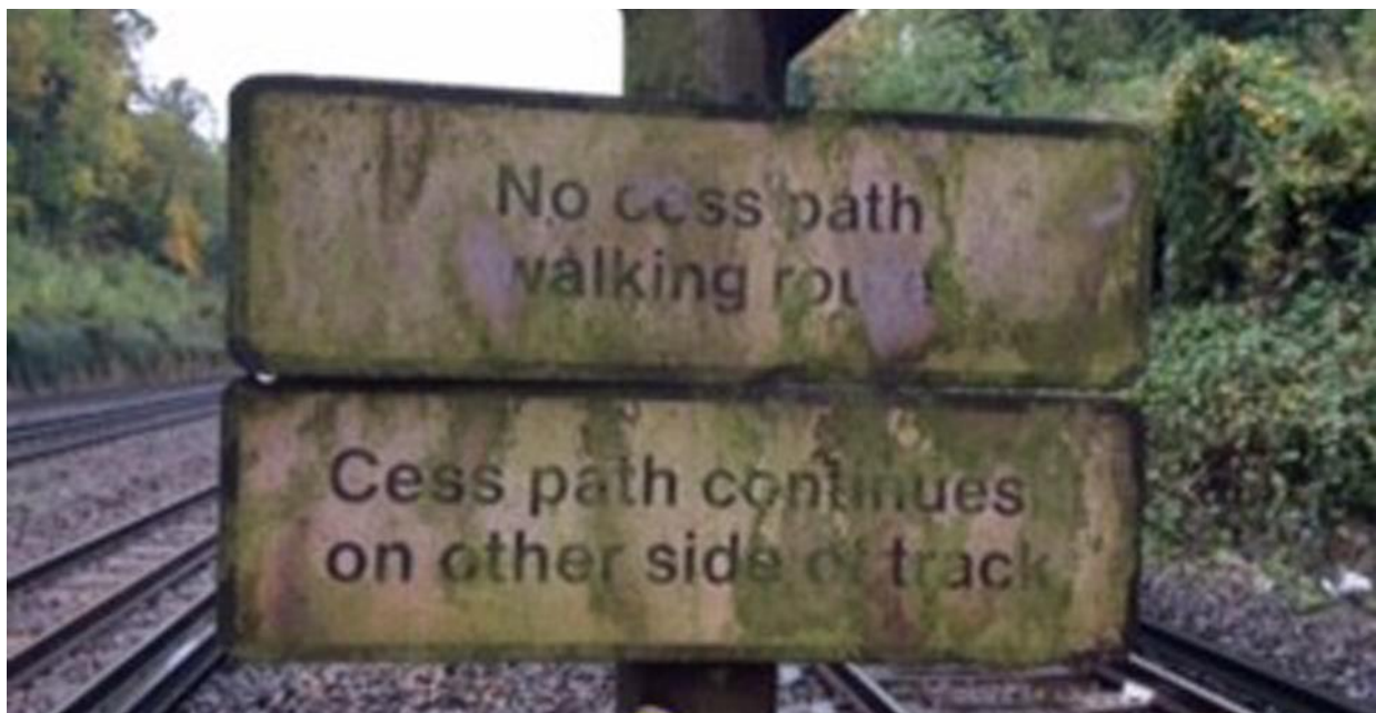
Photograph taken after the incident, showing the sign indicating the limit of the position of safety in the midway (courtesy Network Rail)
