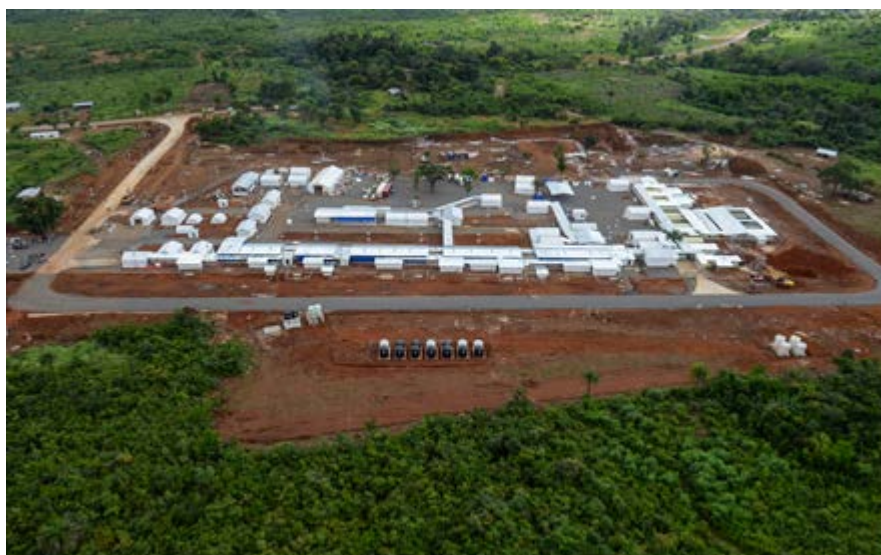
Figure 1: The Kerry Town Treatment Centre in Sierra Leone near the capital Freetown.
