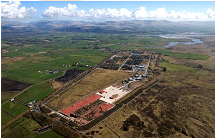
Photograph of the LLWR taken from the North West, Courtesy of LLW Repository Limited
