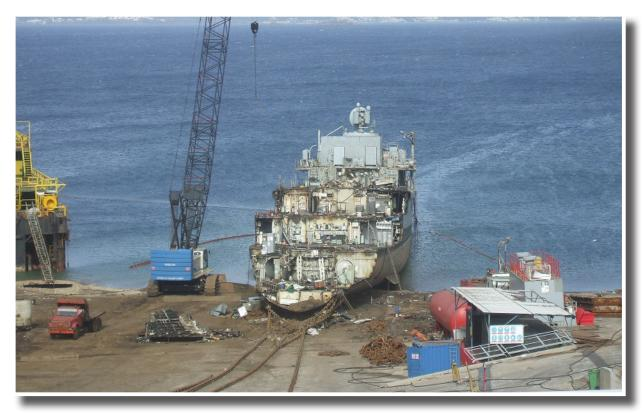
15 Feb 2016 – Ex-HMS York showing the dismantling of the top deck and accommodation. The large blocks removed from the vessel are with the use of heavy lift cranes. Secondry cutting and further processing and material separation takes place.
