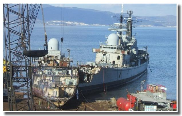
7 Jan 2016 – Ex-HMS Edinburgh in the foreground & Ex-HMS York in the background. Showing stages of pre-cutting ready for the hull to be winched up the dry slipway. Heavy Machinery is used to remove large pieces of the vessel for processing.
