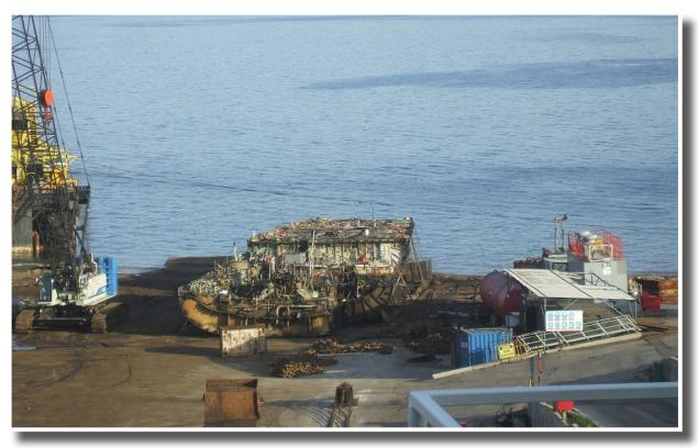
Final dismantling of the pump & engine room. The final recycling of the hull takes place completely on dry land where the remaining part of the keel is winched on to the landing area.
