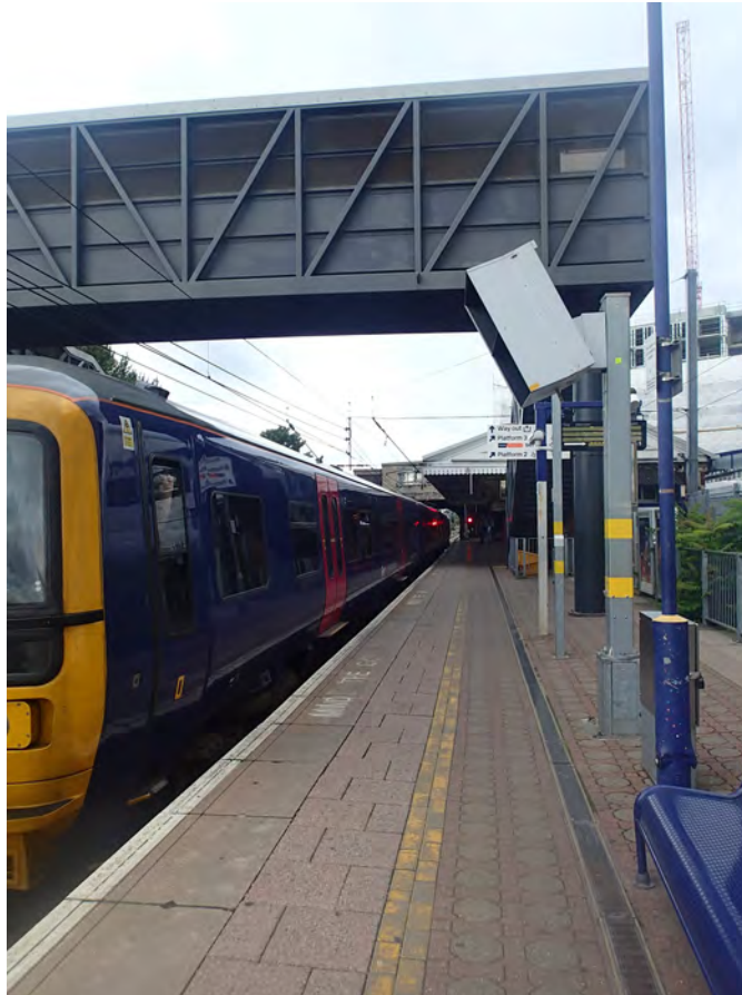
Figure 7: Platform 4 (Up relief line) at Hayes & Harlington
