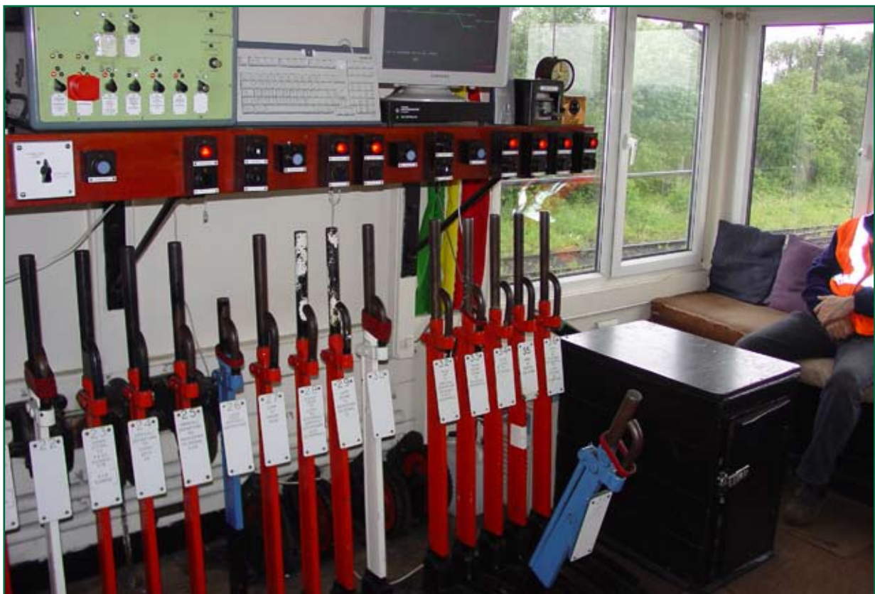
Figure 10: Interior of Maltby Colliery signal box
