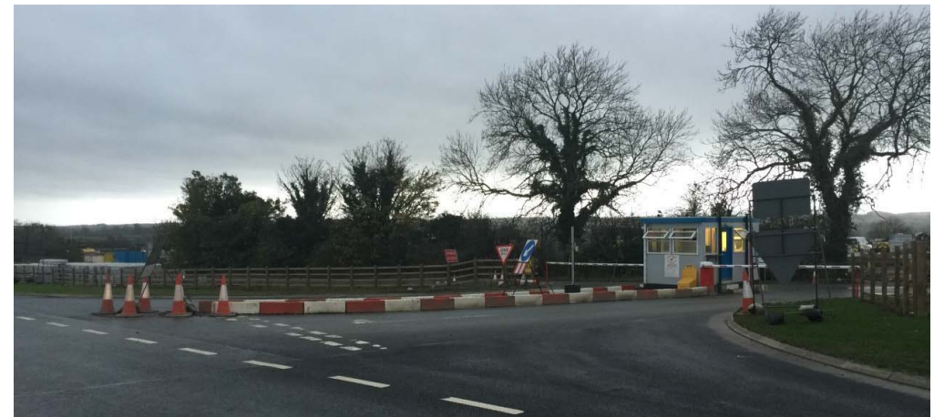
Example of a vehicle site entrance/exit point
