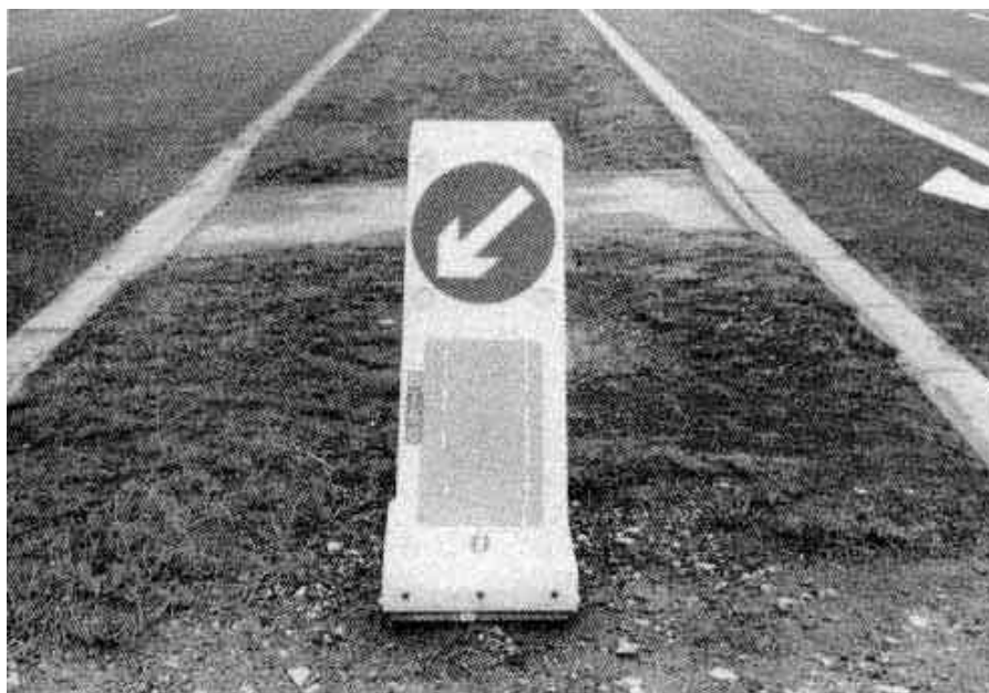
Photograph 2.17-7: Safety Bollard
