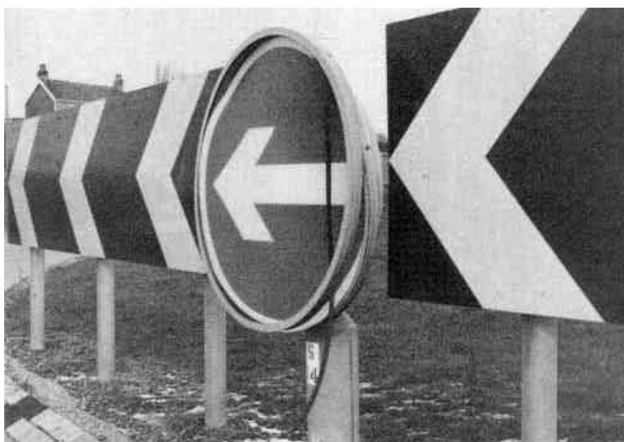
Photograph 3.17-4: COFR - Physical condition of frame
