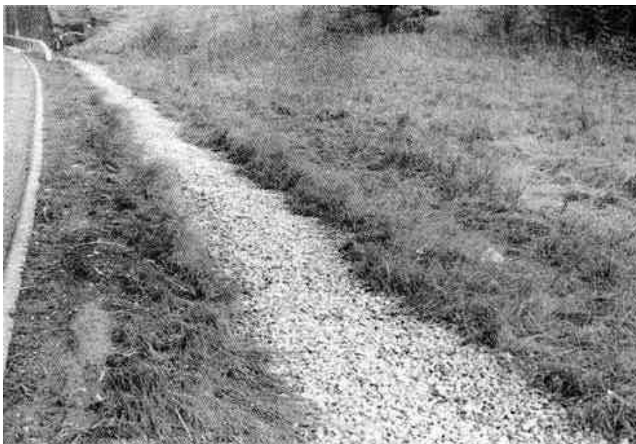
Photograph 2.7-8: Filter Drain
