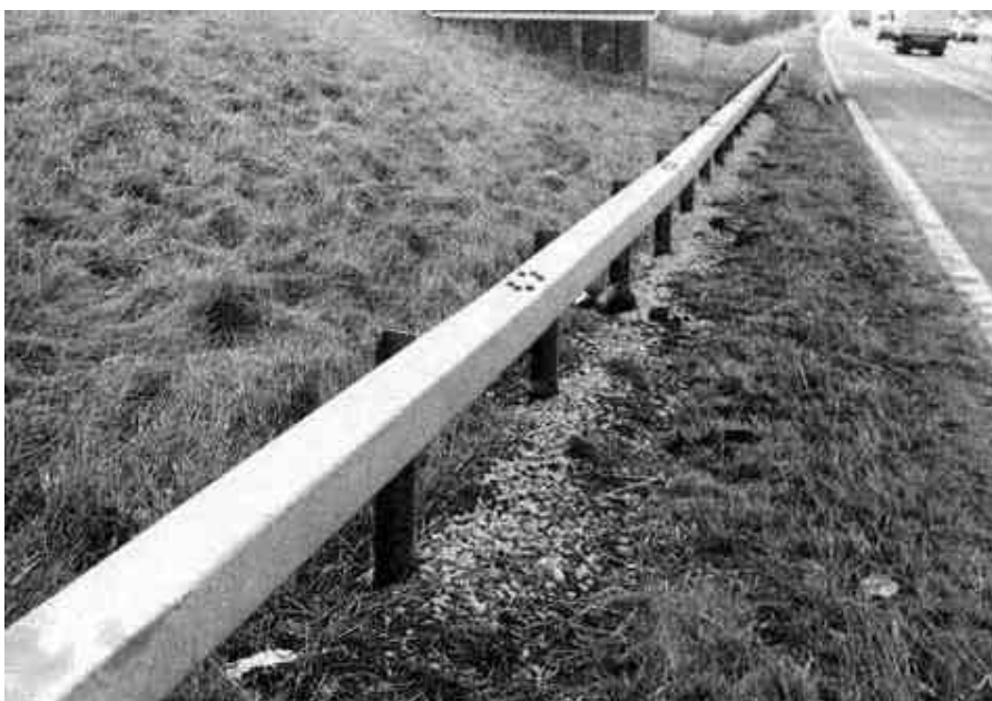
Photograph 2.13-2: Untensioned, Single Sided, Metal, Box Safety Fence
