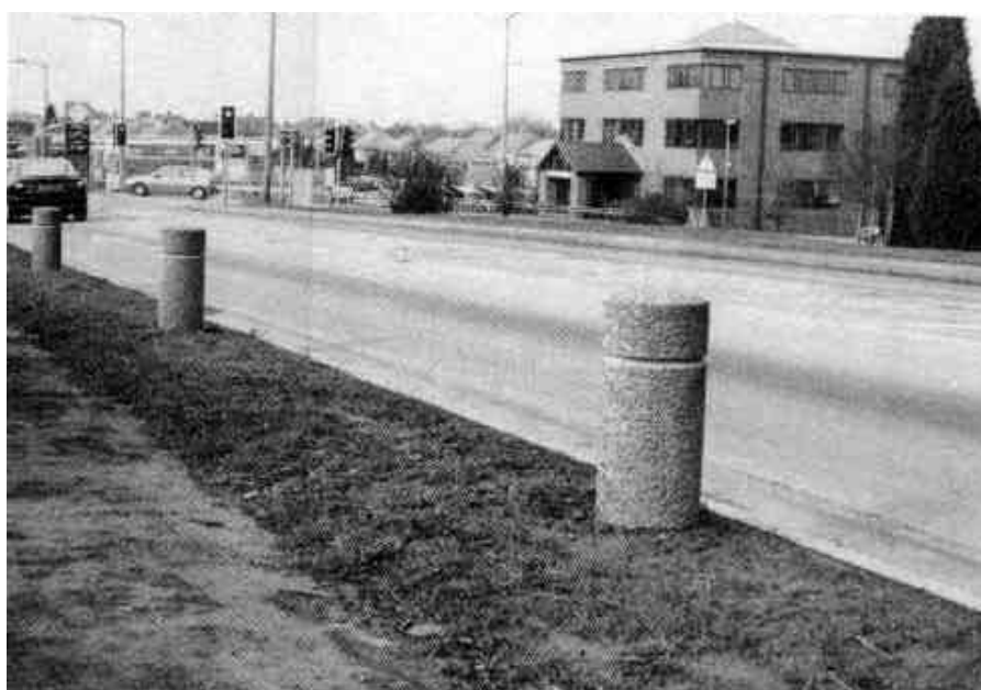
Photograph 2.17-8: Safety Bollard
