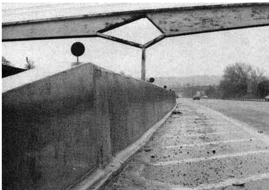
Photograph 2.13-3: Concrete Safety Barrier
