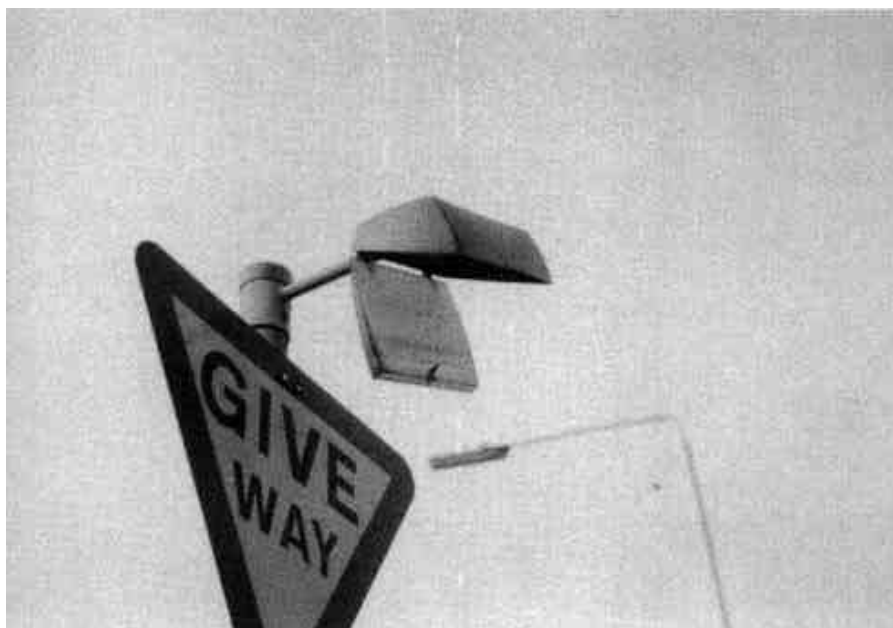
Photograph 3.17-3: COFT - Physical condition of fittings
