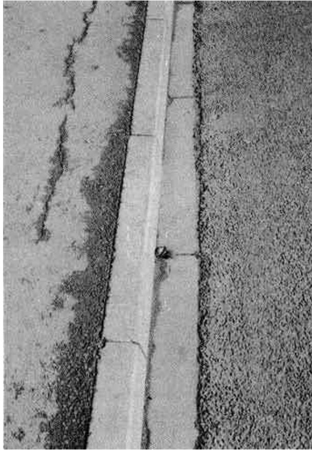
Photograph 2.6-5: Channel - Pre-formed Concrete Blocks
