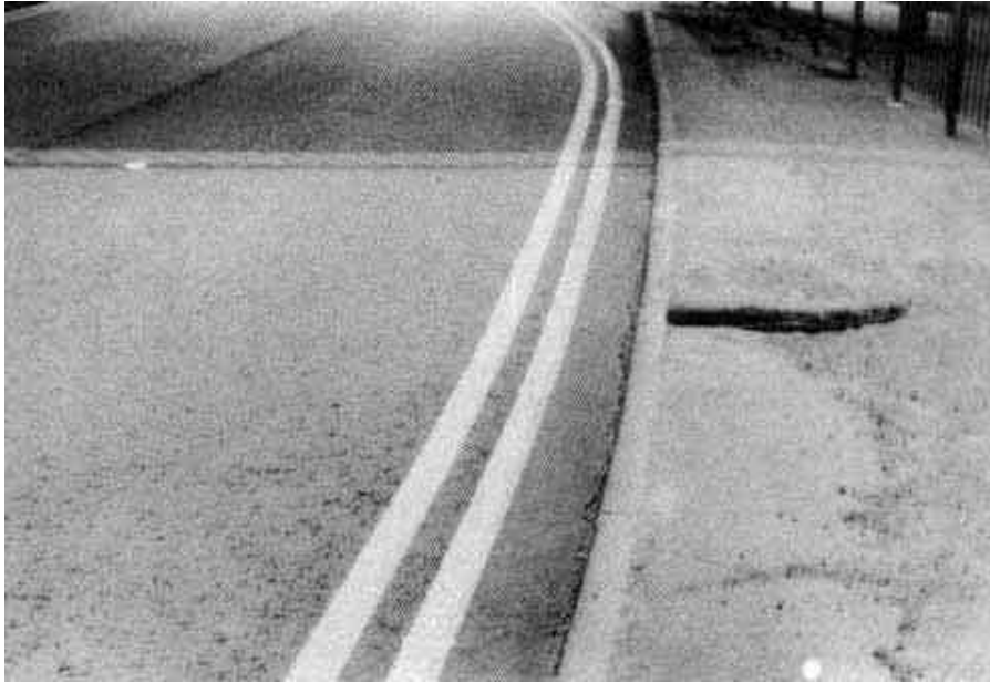
Photograph 2.16-5: Longitudinal Road Markings - Double Yellow
