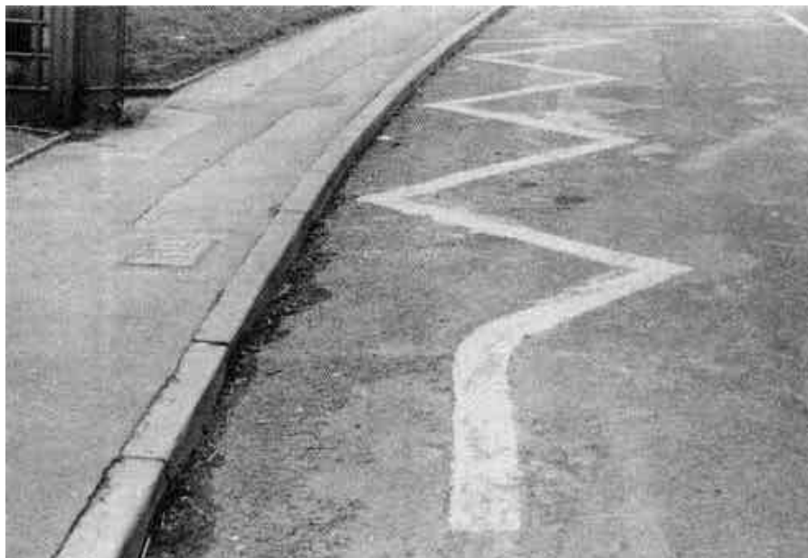
Photograph 2.16-7: Longitudinal Road Markings - Zig-zag
