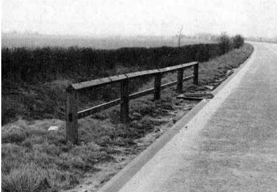
Photograph 2.13-7: Timber Pedestrian Guard Rail
