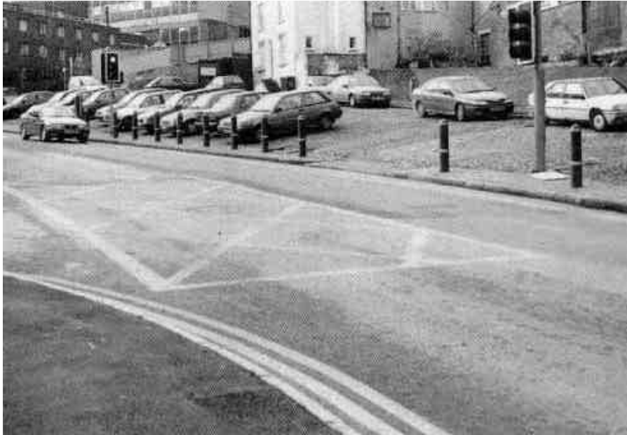
Photograph 2.16-3: Hatched Road Markings - Cross
