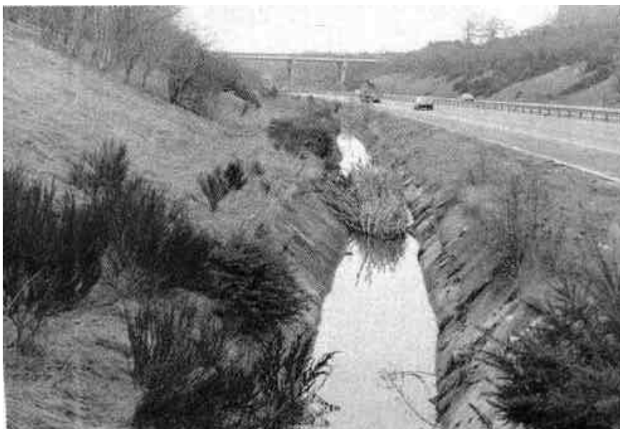
Photograph 2.7-6: Lined Ditch
