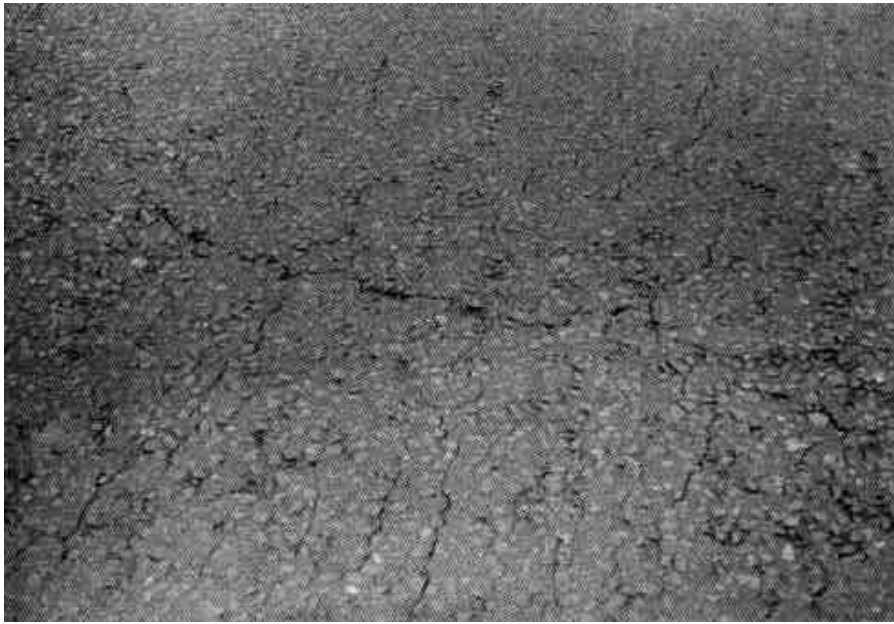
Photograph 3.3.1-1: LOCK - Localised Cracking
