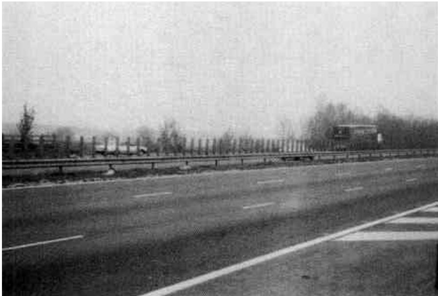
Photograph 2.14-2: Anti-Glare Fencing
