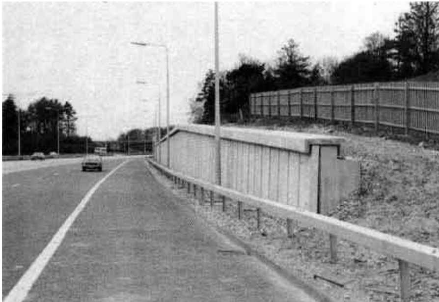
Photograph 2.14-8: Reinforced Concrete Retaining Wall
