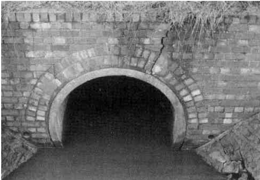
Photograph 3.7.7-2: CRCK - Cracking
