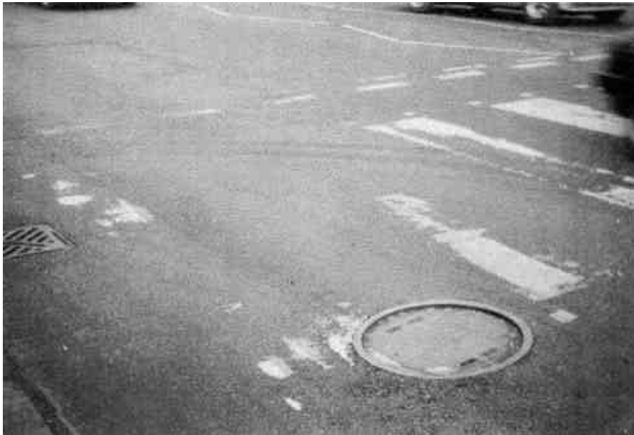
Photograph 3.5-2: ICLV - Difference in component levels
