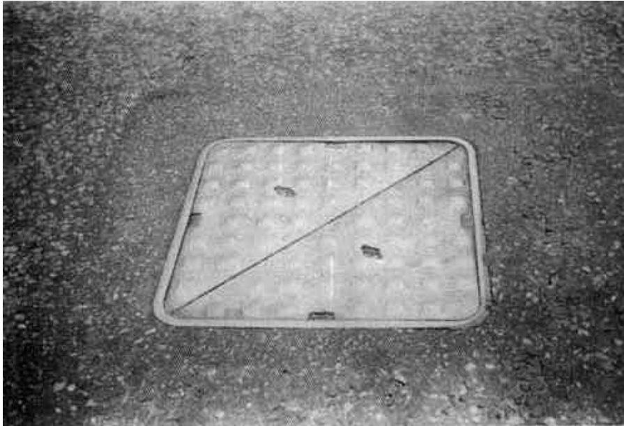
Photograph 3.5-5: SMTH - Smooth surface
