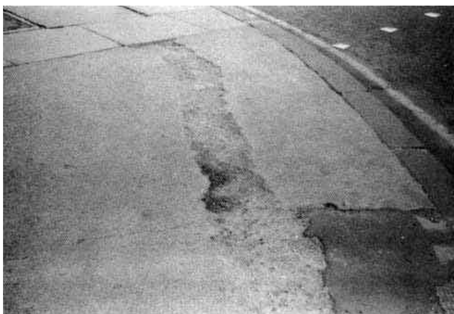
Photograph 3.4-12: RDLV - Trench RI - difference in level
