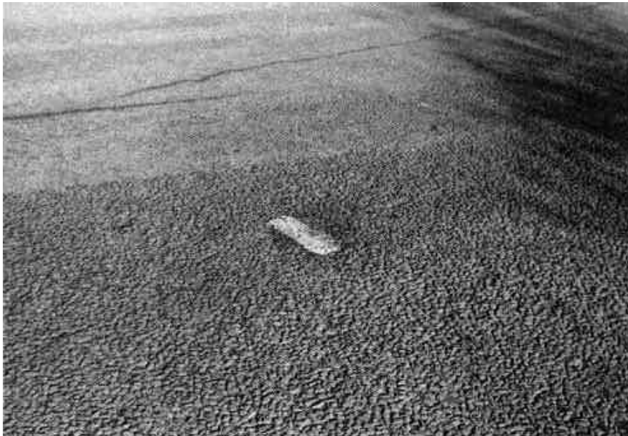
Photograph 2.17-13: Reference Marker Point - Paint Pad
