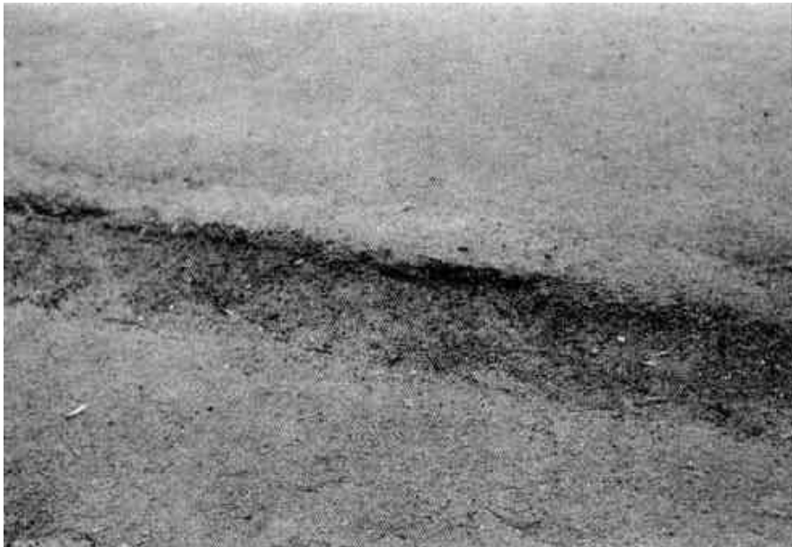
Photograph 3.3.1-10: TDLV - Trench RI - difference in level
