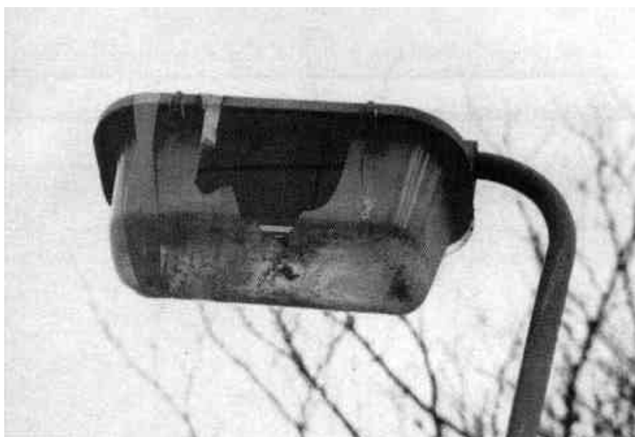
Photograph 3.19-6: COFT - Physical condition of fittings
