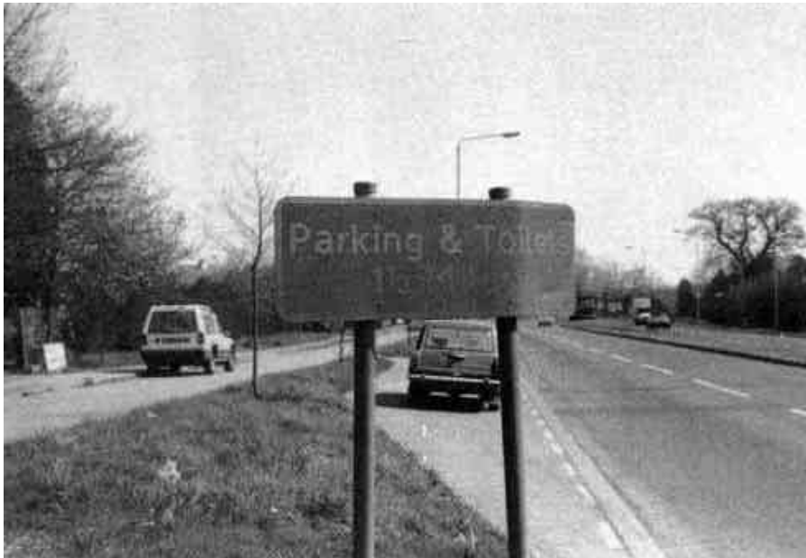
Photograph 3.17-10: DIRT - Dirty sign
