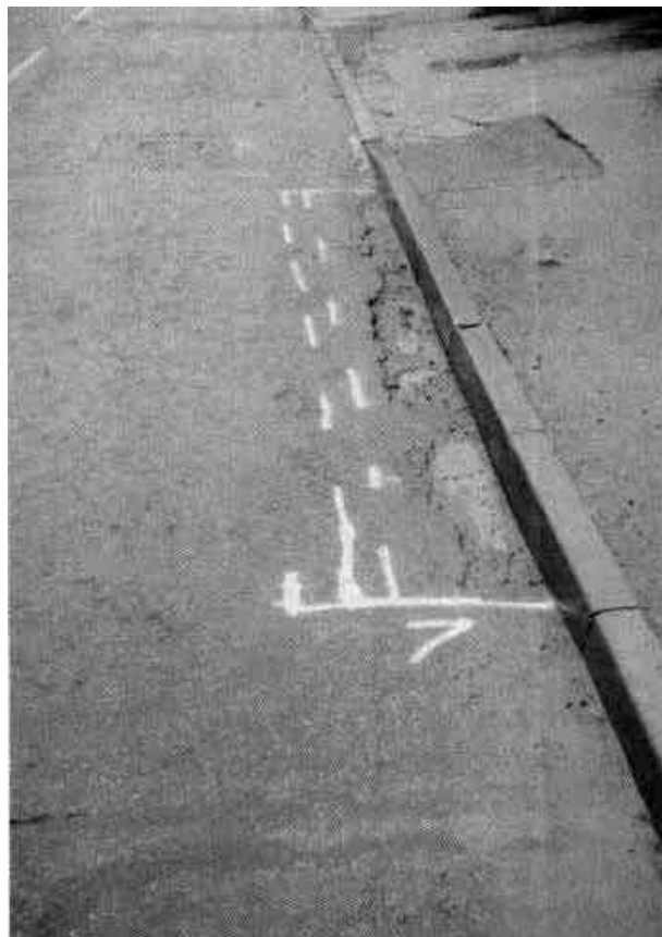
Photograph 3.3.1-1: LOCK - Localised Cracking
