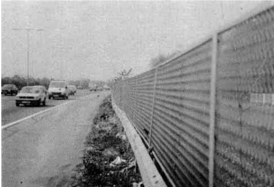
Photograph 2.14-1: Anti-Glare Fencing
