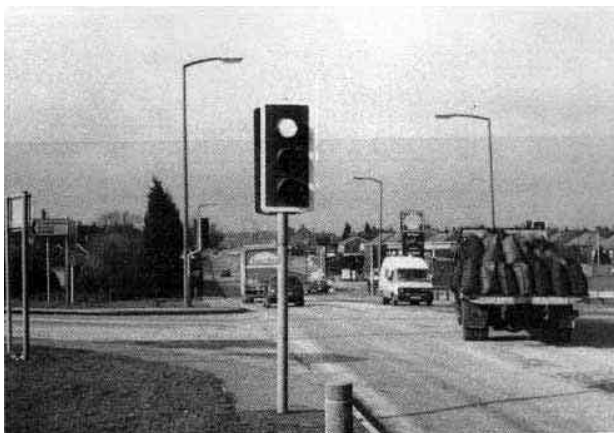
Photograph 2.18-1: Traffic Signals - Traffic Control Junction
