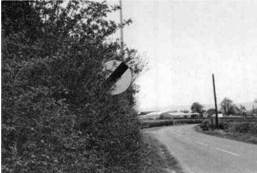
Photograph 3.17-9: OBSG - Obscured sign
