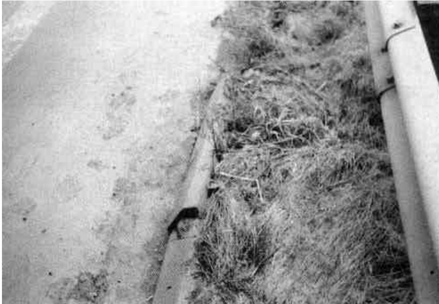
Photograph 3.6-1: EVPJ - Vertical projection > 20mm
