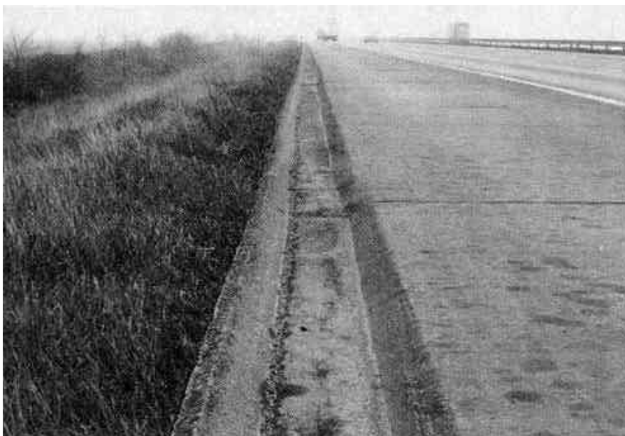
Photograph 2.6-4: Channel - Continuous Concrete
