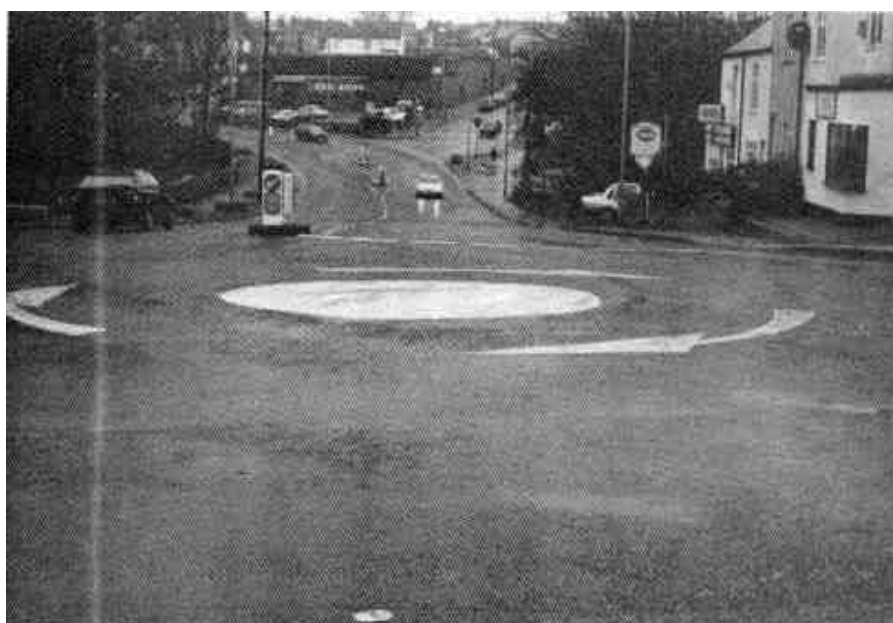
Photograph 2.16-12: Transverse and Special Road Markings - Roundabout
