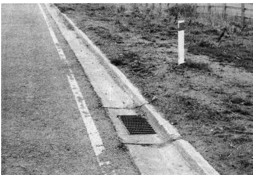
Photograph 2.6-8: Combined Kerb and Channel
