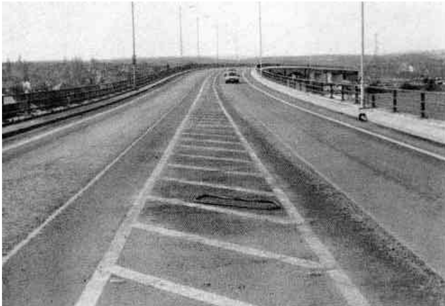
Photograph 2.16-1: Hatched Road Markings - Diagonal
