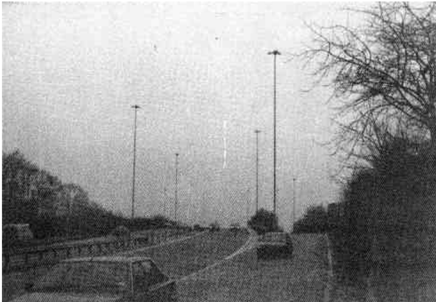
Photograph 2.19-2: High Mast Column
