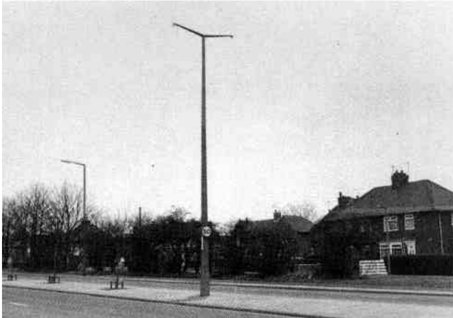
Photograph 2.19-1: Double Mounting (Foreground) Single Mounting (Background)
