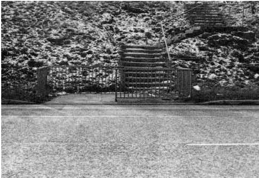
Photograph 2.13-6: Pedestrian Guard Rail
