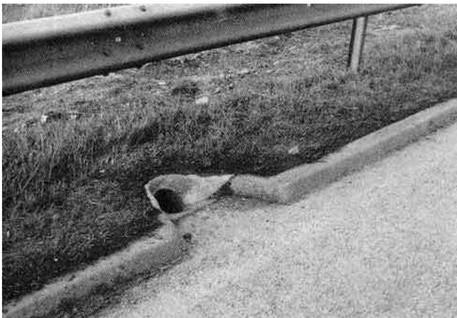
Photograph 2.7-4: Piped Grip
