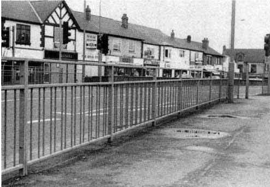
Photograph 2.13-5: Pedestrian Guard Rail
