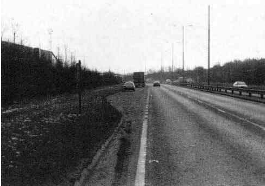
Photograph 3.17-13: RWAY - Pointing wrong way
