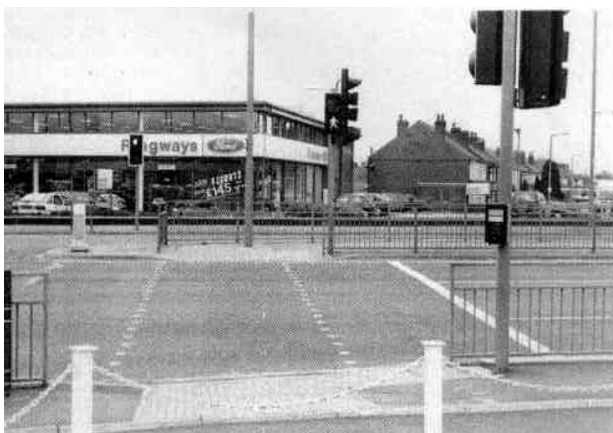
Photograph 2.18-2: Pedestrian Crossing - Pelican (And Traffic Signals - Pelican)
