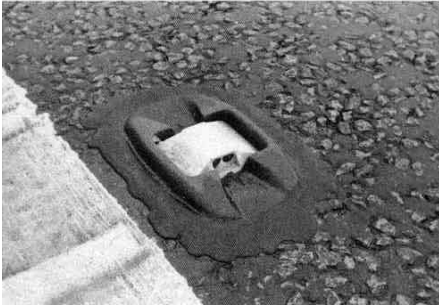
Photograph 2.15-1: Depressible Catseye road stud
