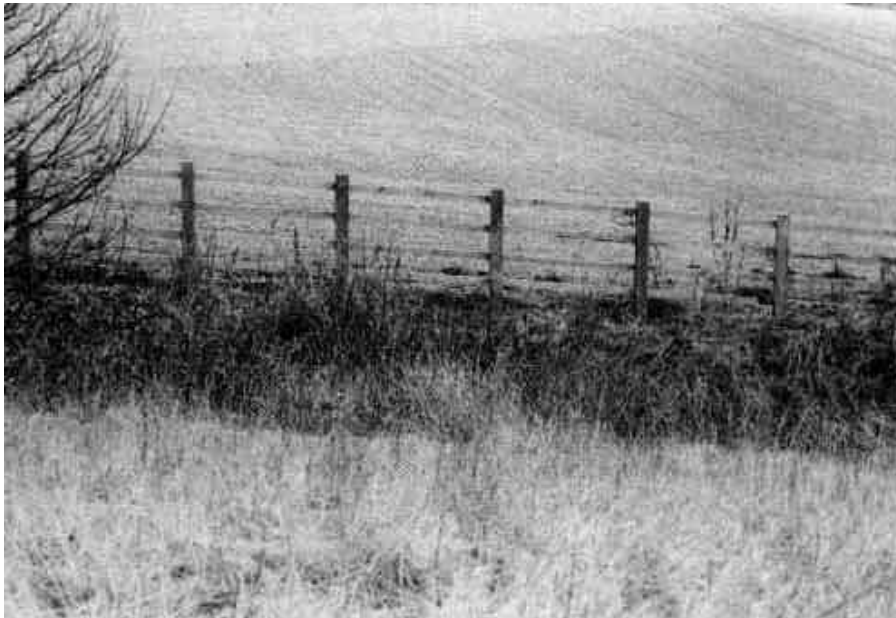
Photograph 2.14-6: Wood Boundary Fence
