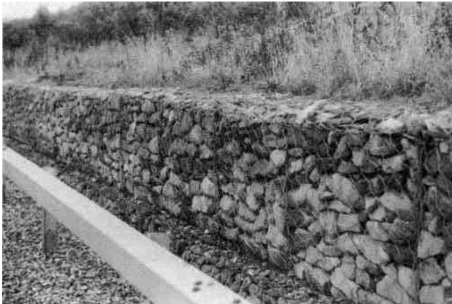
Photograph 2.14-10: Gabion (OTHER) Retaining Wall
