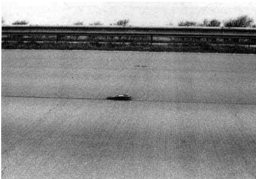
Photograph 3.15-5: MISC - Missing Catseye (NB. displaced catseyes should be removed immediately)
