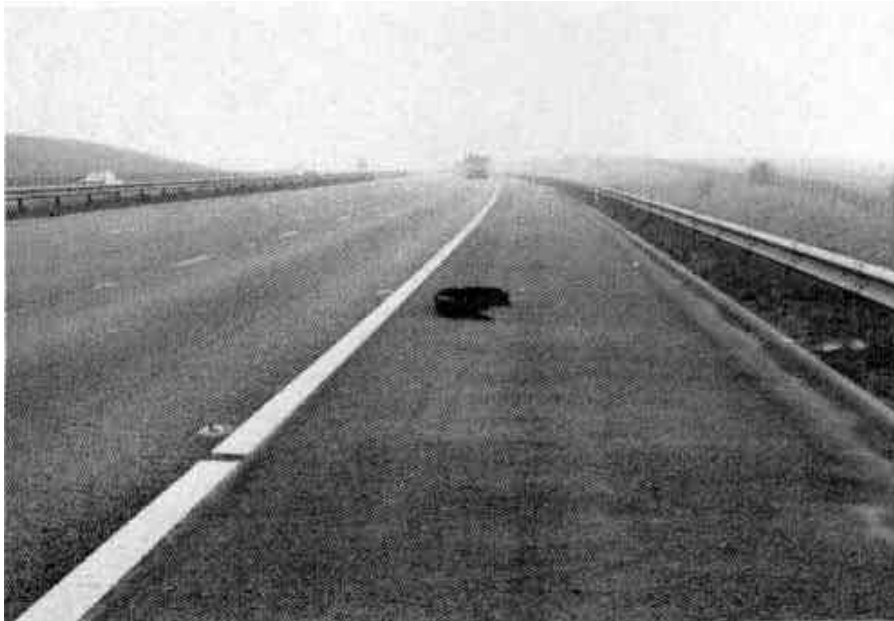
Photograph 3.12-3: DBHS - Debris in hard shoulder
