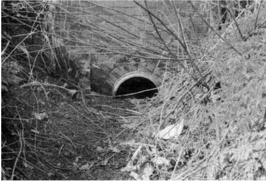
Photograph 3.7.1-1: BLOK - Blockage
