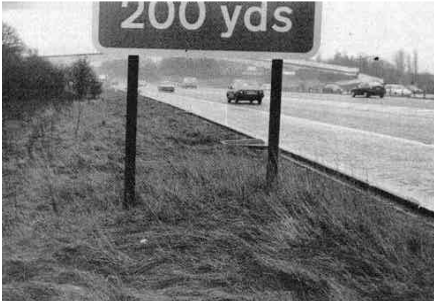
Photograph 2.10-1: Obstacle to mowing
