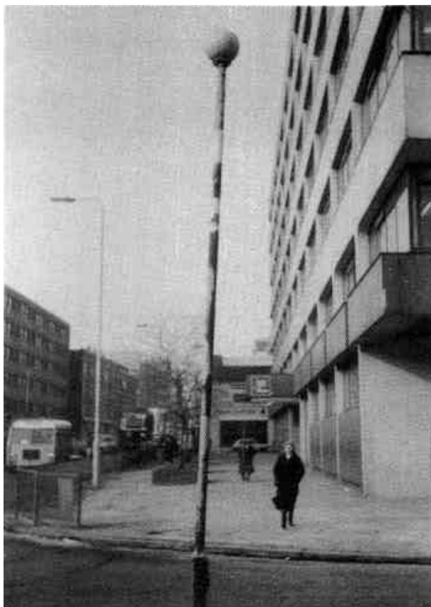
Photograph 3.19-5: LOPT - Loss of surface paint
