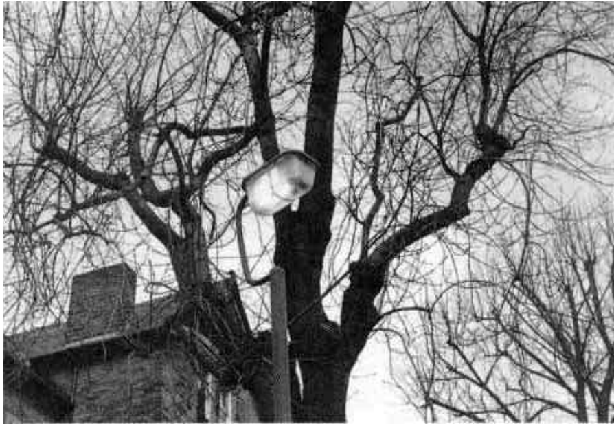
Photograph 3.19-1: LPON - Lamp on during day
