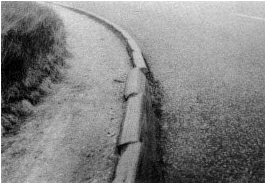
Photograph 3.6-2: EHPJ - Horizontal projection > 20mm
