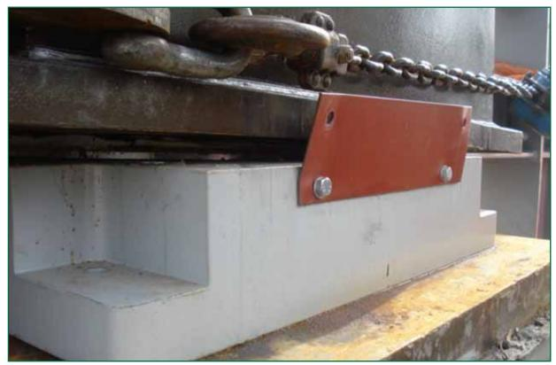
Figure 23: Failed transit cleat on south-east bearing (photograph BB-CJV)
