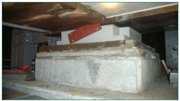
Figure 22: South-east bearing following collapse showing a failed transit cleat.
