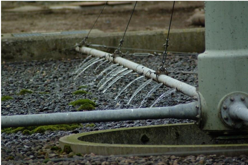
Figure 8 Cokermonth WwTW- a site with planned development due to supply demand reassessment.
