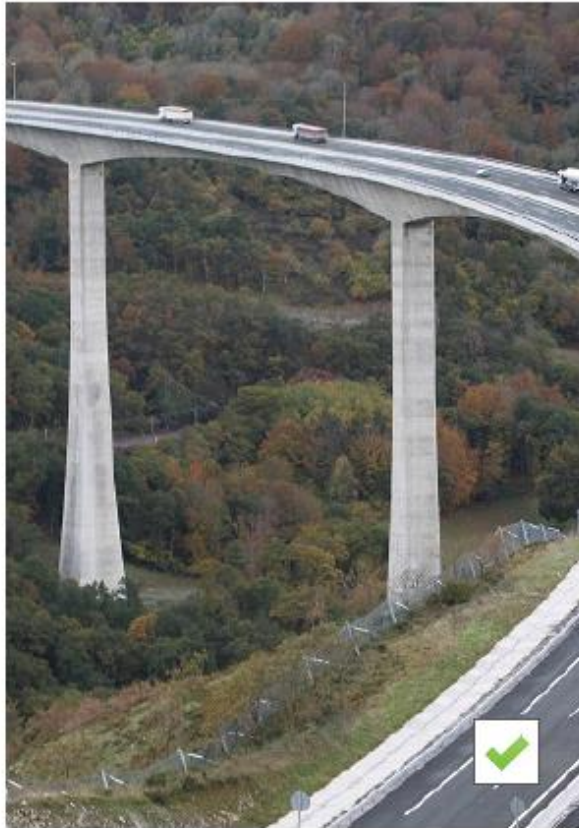
Elegant concrete piers: piers and deck structure designed as one coherent system, © Ferrovia
