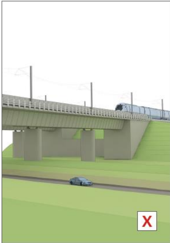
Poor abutment design: substantial concrete abutments and retaining walls, © Grimshaw
