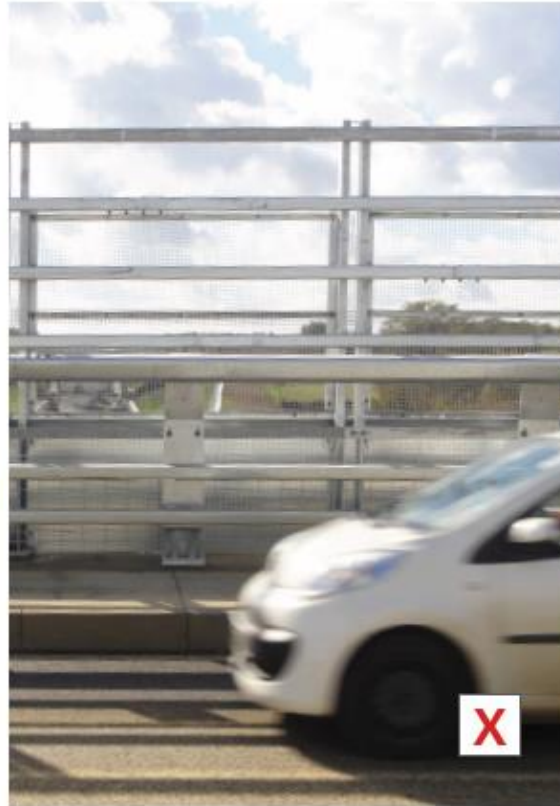
Closer view of H4a barriers plus pedestrian barrier and additional higher protection above track / OHLE, © Grimshaw
