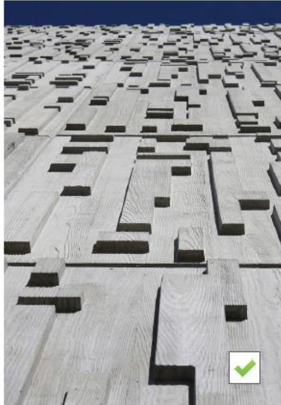
Precast concrete retaining walls: potential for texture and pattern in pre-cast panels, © Glen Waverley / urban.melbourne
