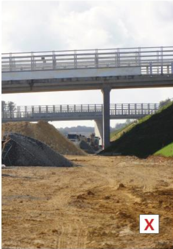
Visual impact of H4a barriers plus pedestrian barrier and additional higher protection above track / OHLE, © Grimshaw
