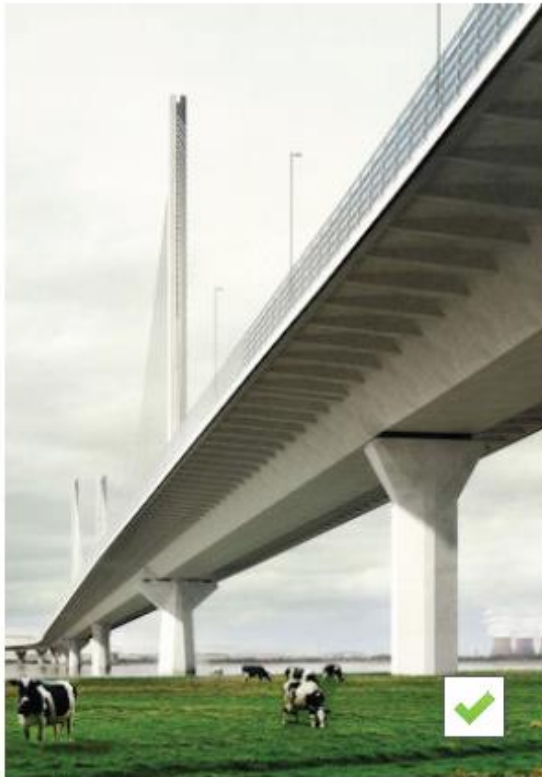
Precast concrete deck edge: deck spine beam is cast into shadow, © merseygateway
