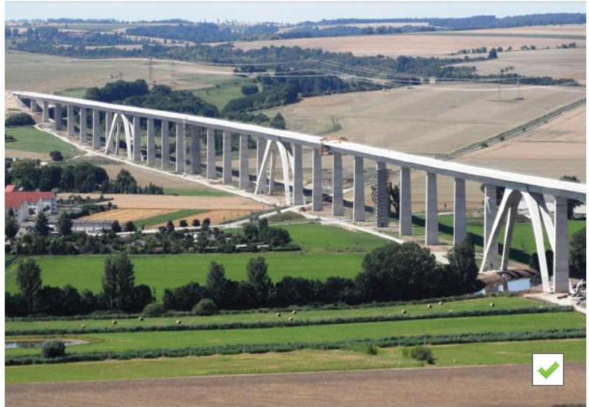
Pier functions expressed in design: slim integral piers with special piers to resolve braking and bracing forces, © Holger Althaus / SBP
