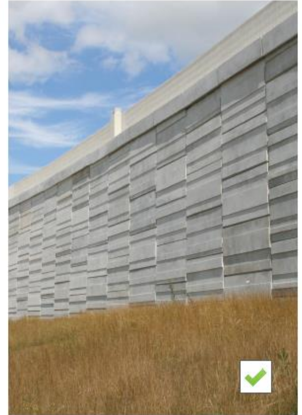
Reinforced earth wall: potential for texture and pattern in pre-cast panels, © Prekast Beton
