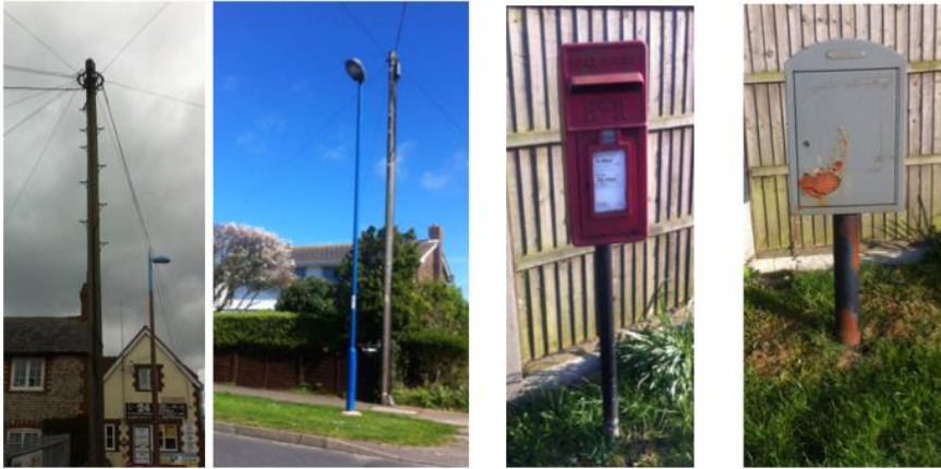
Figure 7 Other poles found near roads e.g. telecom, energy, streetlights and postal boxes.
