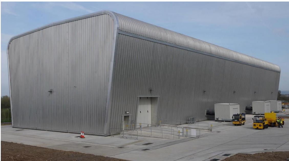
Figure 7-4 Interim Storage Facility for ILW (Courtesy Magnox Ltd)
