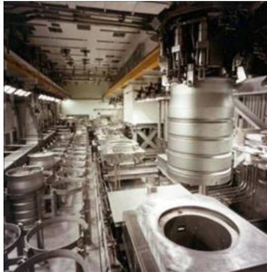
Figure 7-3 Magnox Waste Encapsulation Plant (Courtesy Sellafield Ltd) with Unshielded Waste Package
