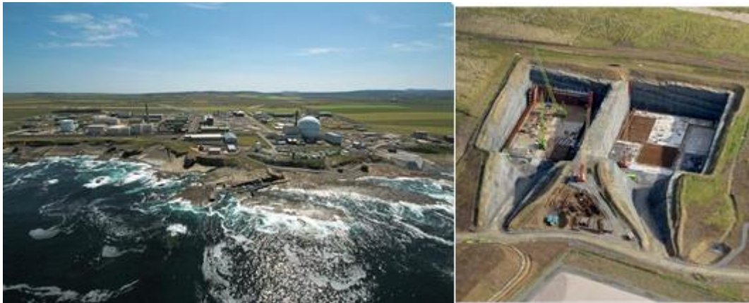
Figure 4-5 Dounreay Site. Partial view of the site on the left showing the DFR sphere, near-surface disposal facility under construction on the right (Courtesy Dounreay and NDA)
