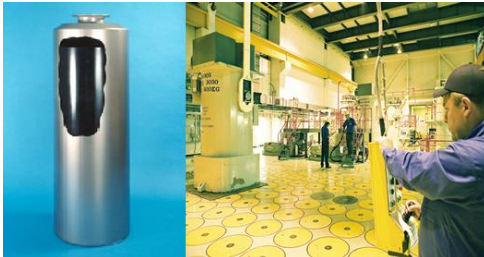
Figure 7-1 Cut-away Vitrified HLW canister (Left) and Vitrified Product store, Sellafield (Right) (Courtesy Sellafield Ltd)
