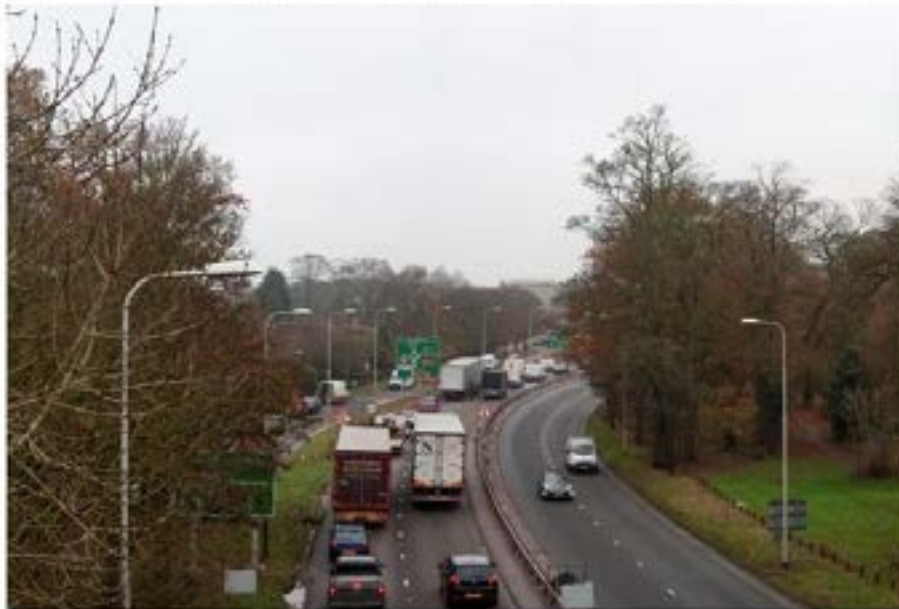
The current A38 approaching Markeaton Island
