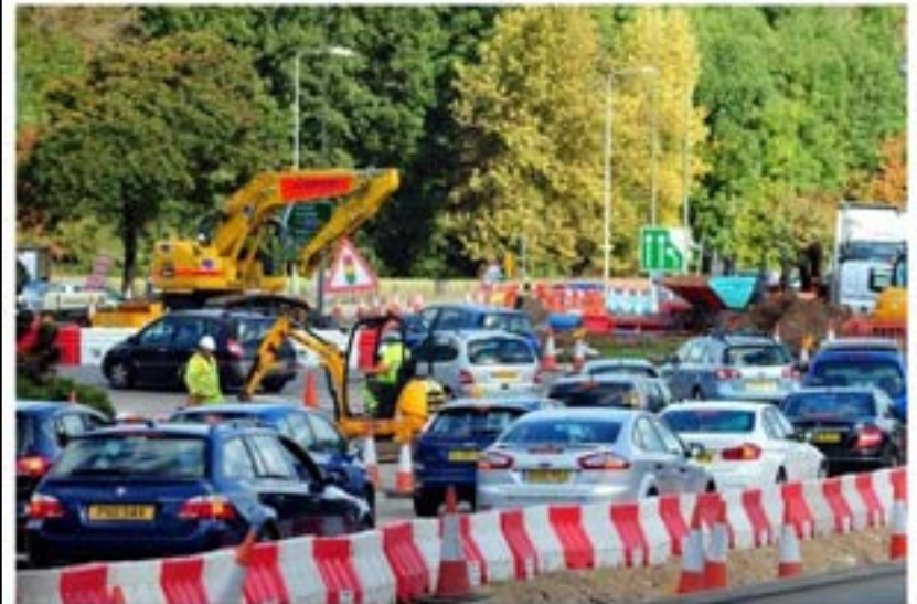
Congestion amid the Markeston Island roadworks last autumn.
